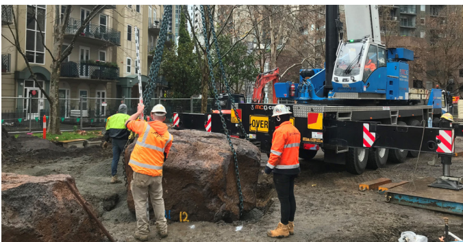
20 ton rocks being installed between Kavanagh Street and Moore Street
