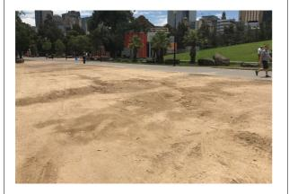
**Incident:** Heavy vehicle movement and heavy infrastructure placement through the site when wet.
