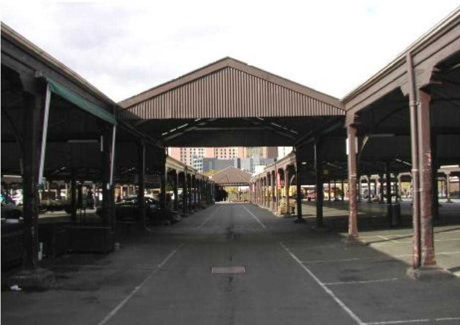
Figure 58 Typical post detail and 1920s covered way, A-E Sheds
