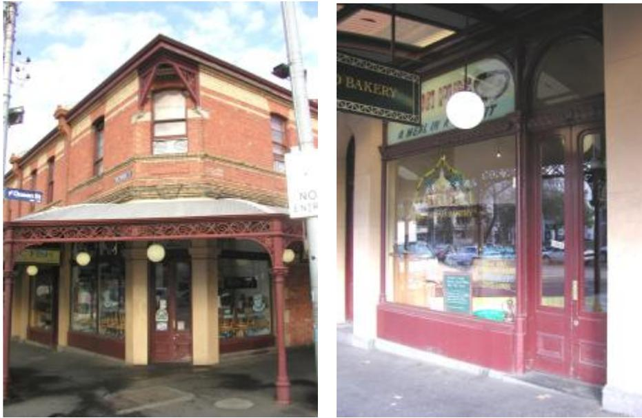
Figure 39 Splayed north-west corner (left) and typical shopfront (right)
