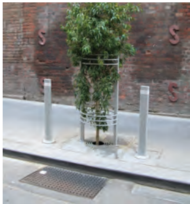
Water sensitive tree pit collects storm water from Little Collins Street, Melbourne.
