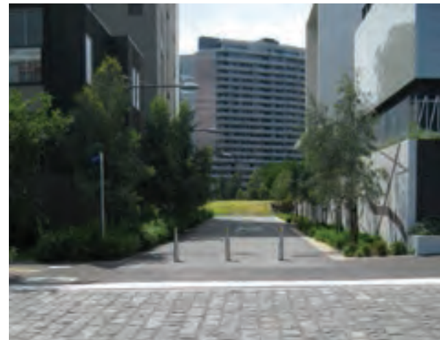
Safe laneway connection between Victoria Green and Docklands Park is well lit and addressed by residential building entries.
