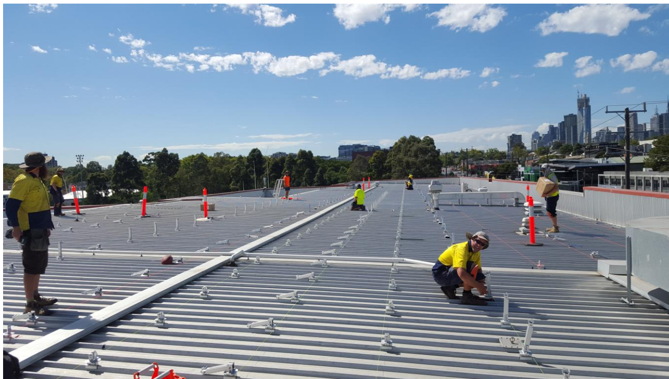
Workmen installing the 200kW system
