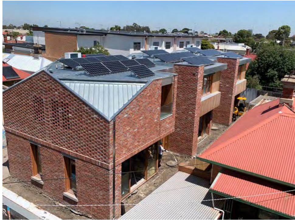
Solar PV installed on the Davison Collaborative. Image by Guy de Vos
