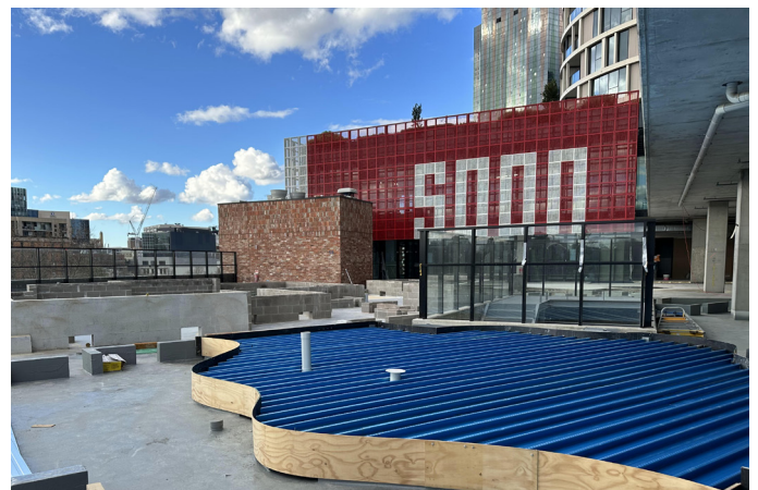
Landscaping and waterproofing works on the rooftop terrace
