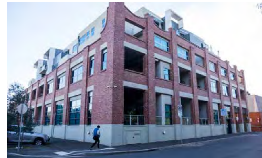
Figure 7: Raised floor level in flood risk area
