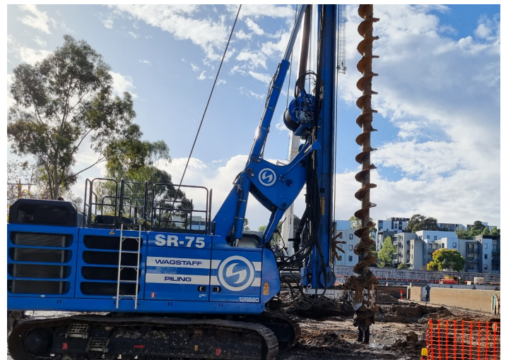
Piling will continue over the coming months
