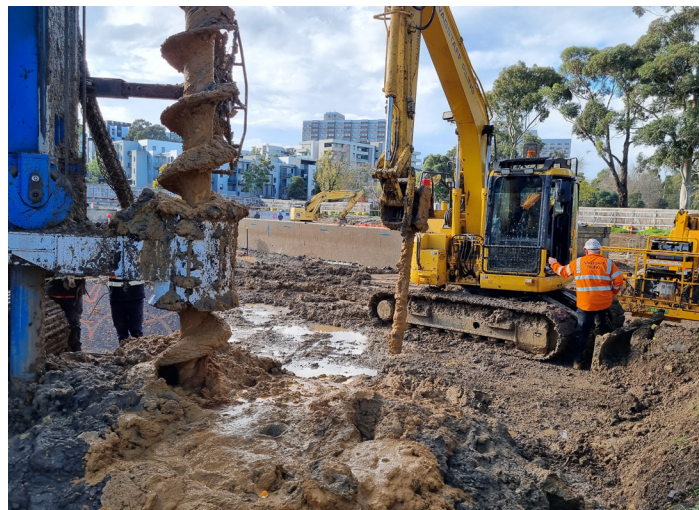
Backfilling is now complete
