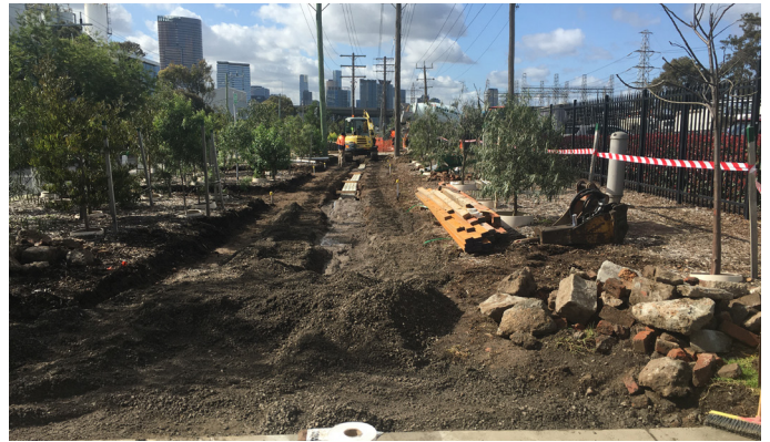
Gateway to GMH excavation works
