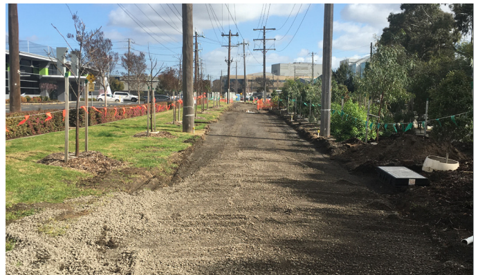
Gateway to GMH footpath excavation works
