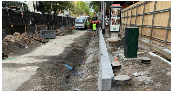
Construction of kerb and drainage works underway
