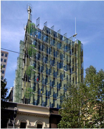
Figure 2. Image of the future façade CH2
