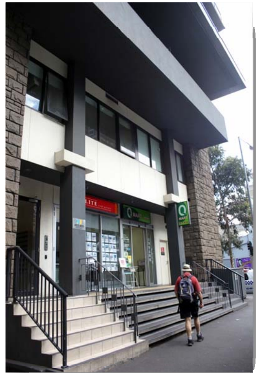
• Figure 132 453-457 Elizabeth Street, ground level
