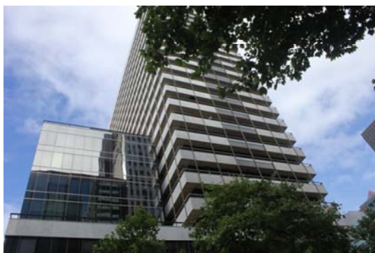
• Figure 83 435-455 Collins Street from south-east, showing south addition
