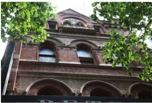
• Figure 56 upper level facade
