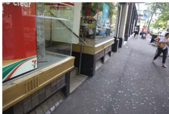
• Figure 155 104-110 Exhibition Street, west ground level: shopfront plinths and basement lights
