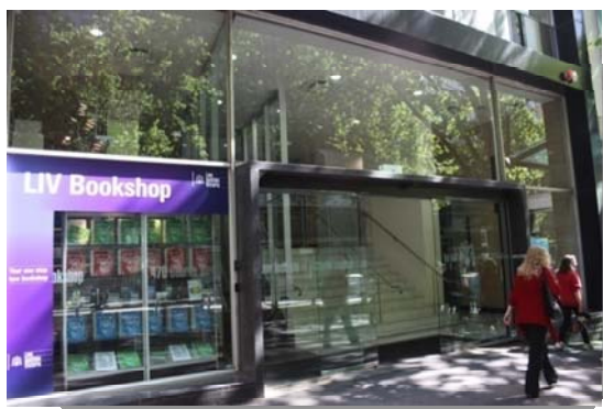
• Figure 60 ground level entry
