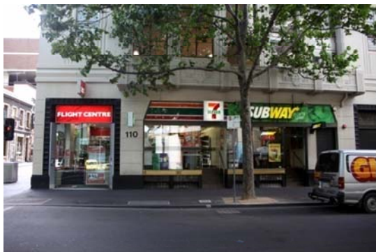
• Figure 154 104-110 Exhibition Street, ground level west face.
