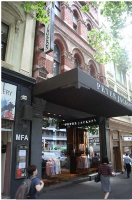
• Figure 55 418-420 Bourke Street lower facade
