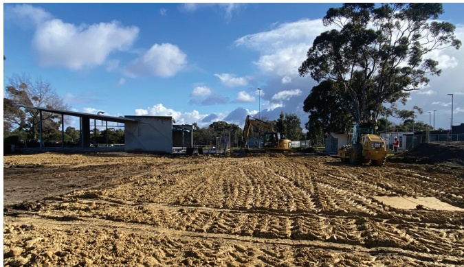
Demolition of the old pavilion is now complete
