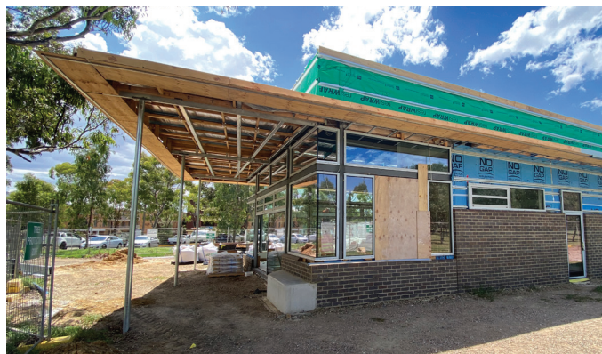
The exterior brick work has been completed
