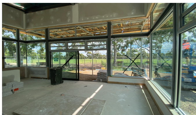
Windows have been installed
