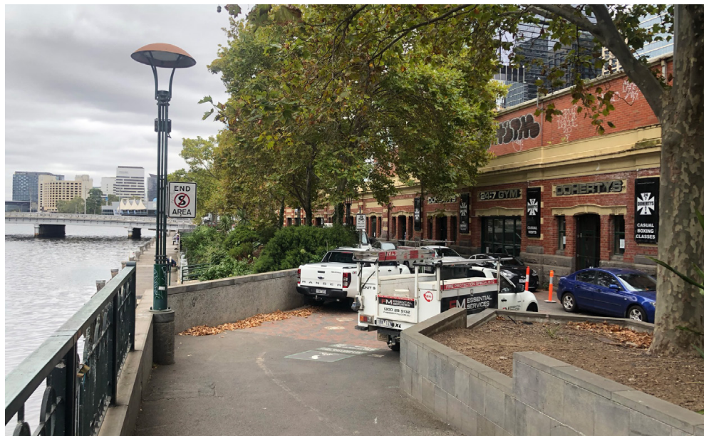
Banana Alley existing conditions
