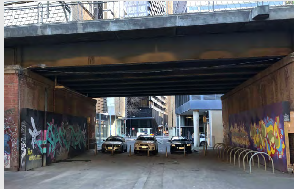
Existing condition beneath railway viaduct at Rebecca Walk (River Park Precinct)
