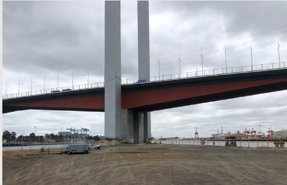
Existing view towards Bolte Bridge from North Wharf (Saltwater Wharf Precinct)
