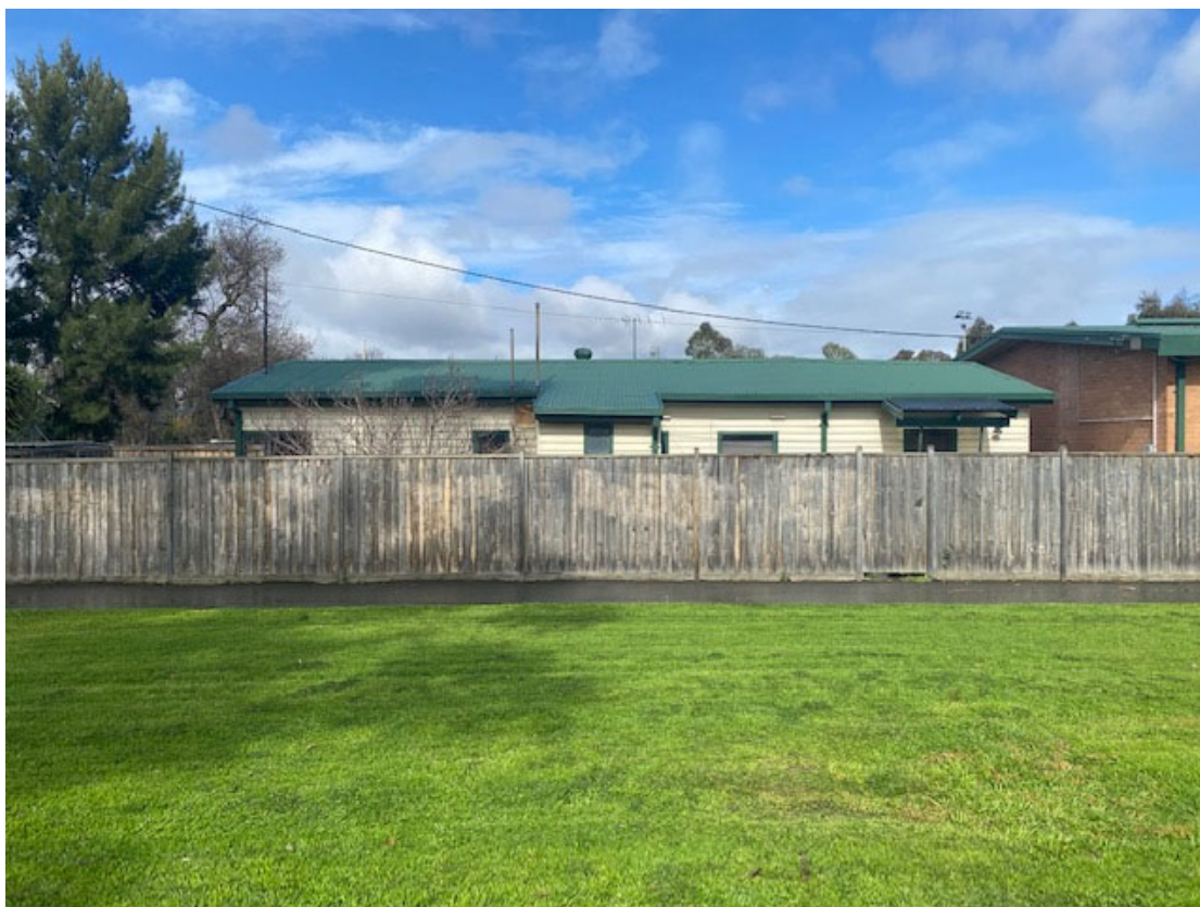
Figure 4: Site Photograph from the north (Source: City of Melbourne)
