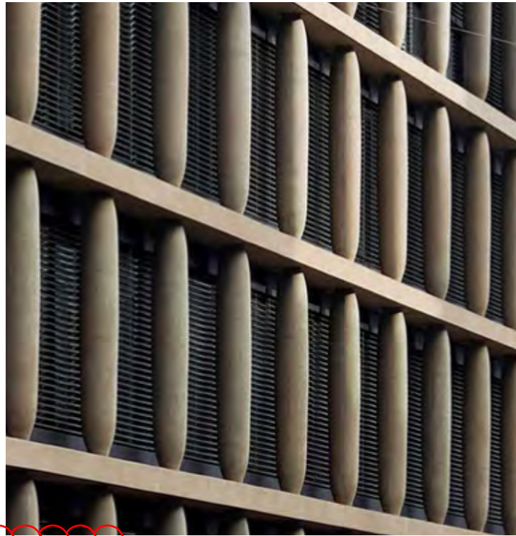
E.PNE-01 NATURAL CONCRETE COLUMNS/SLAB EDGE
