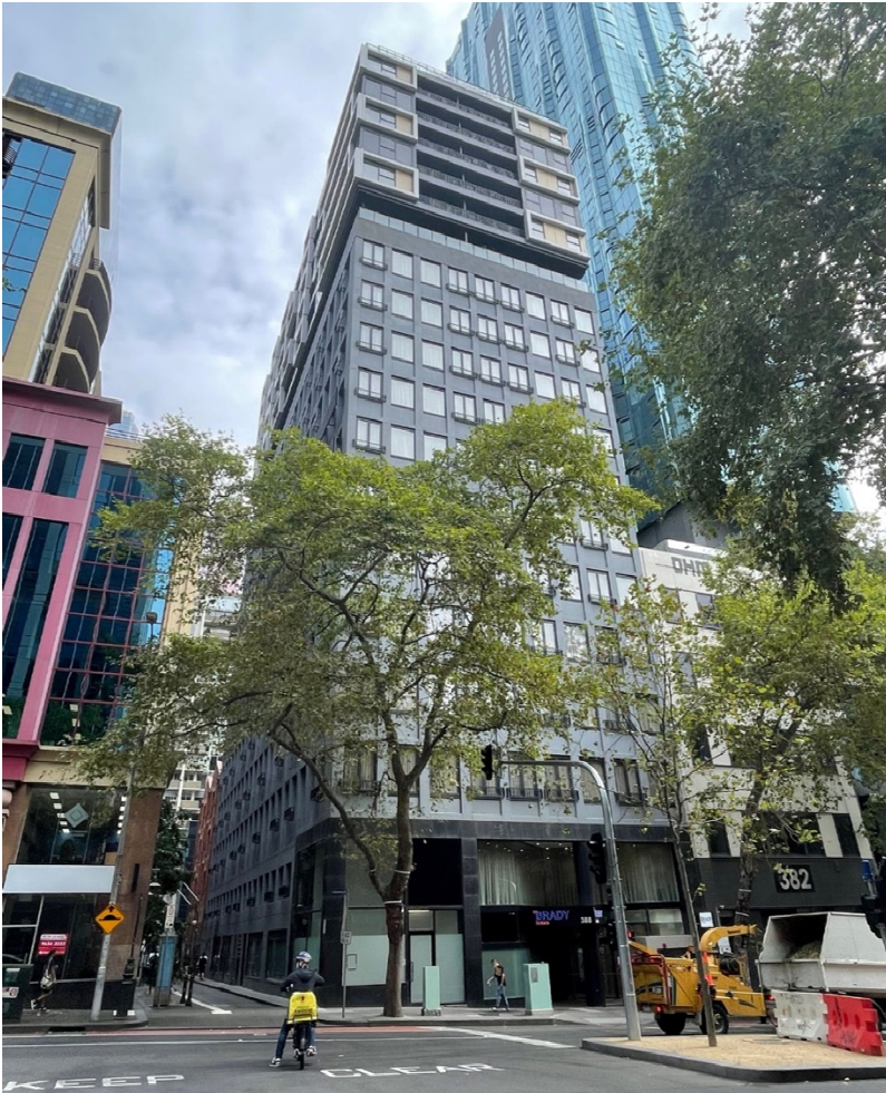
Figure 3 - Photo of site from Lonsdale Street. Taken on 21 February 2022
