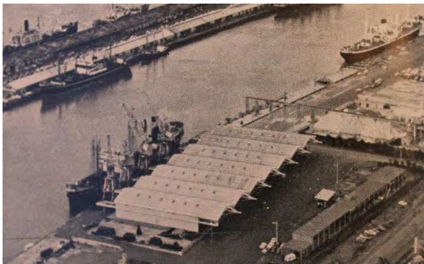
Figure 6: 21 South Wharf including the amenities and office block in c1962 (PMQ January-March 1963 p.32).
