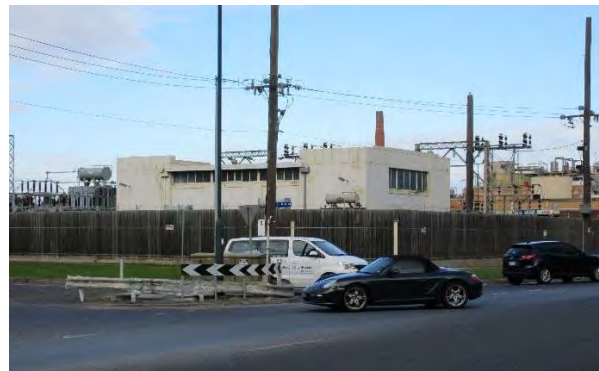
Figure 3: View of the substation from the corner of Salmon and Turner Streets (H Lardner 09/07/2018)
