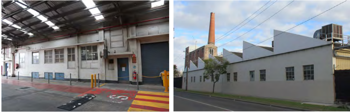
Figures 30 & 31: The west facade of the workshop building from under the covered way, and the sawtooth roof profile of east facade of the workshop building from Douglas Street. (P Mills 4/11/2020; H Lardner 10/07/2018)
