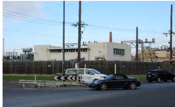
Figure 3: View of the substation from the corner of Salmon and Turner Streets (H Lardner 09/07/2018)
