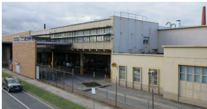
Figure 2: View from Salmon Street (H Lardner 10/07/2018)
