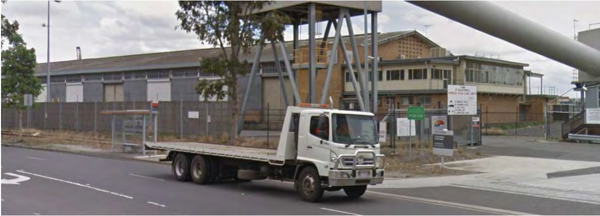
Figure 10: Shed 27, South Wharf at 641-713 Lorimer Street, Port Melbourne (Google imagery Dec 2017)
