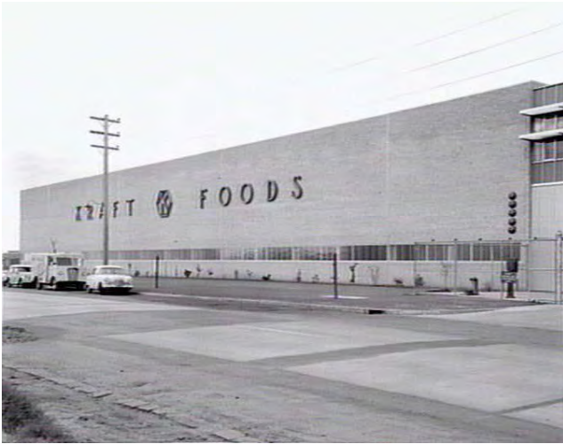
Figure 12: The west side of the production building with large expanse of brickwork broken by a continuous strip window, c1957. This was soon to be obscured by the 1961-62 addition of a covered loading area (SLV, Acc. No. a42751)
