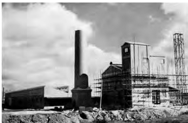
Figure 5: Captioned 'a Victorian dehydration factory' this is the Fishermans Bend boiler house under construction in 1943, with the sawtooth roof of the dehydration factory building behind (Allied Works Council, 1943, p.73).
