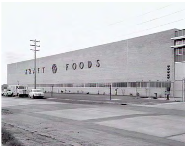
Figure 12: The west side of the production building with large expanse of brickwork broken by a continuous strip window, c1957. This was soon to be obscured by the 1961-62 addition of a covered loading area (SLV, Acc. No. a42751)
