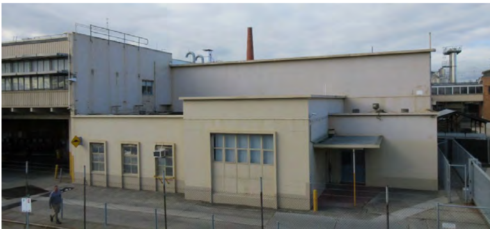
Figures 22: The 1952 yeast/Vegemite factory, including a single storey section seen from Salmon Street which is now used for archive storage. The elevated walkway is on the right. (H Lardner 10/07/2018)
