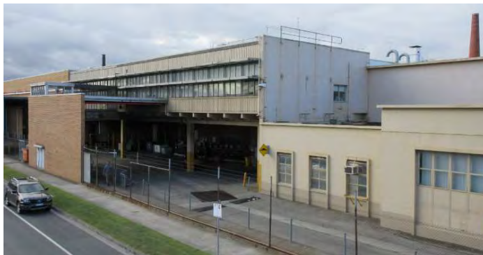
Figure 2: View from Salmon Street (H Lardner 10/07/2018)
