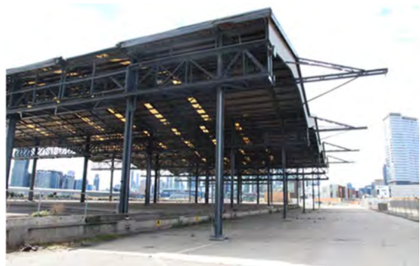
Figure 3: View from south-west showing road alignment and extension past the building. (P Mills, 03/04/2018)
