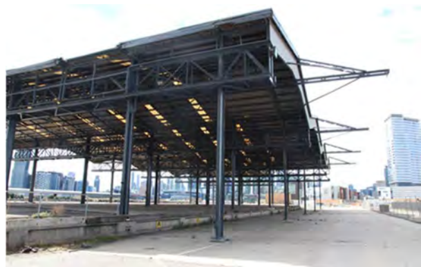
Figure 3: View from south-west showing road alignment and extension past the building. (P Mills, 03/04/2018)
