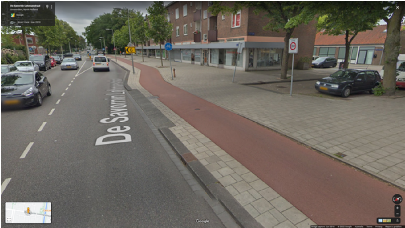
Continuous footpath and bike lane at a side street
