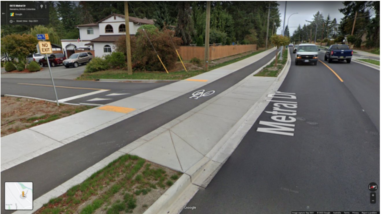
Continuous footpath and bike lane at a side street in Nanaimo, Canada
