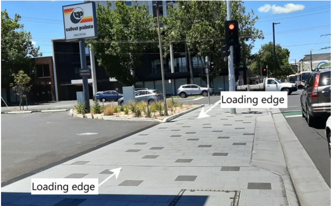
Loading edges visible on continuous footpath on Atherton Rd in Oakleigh
