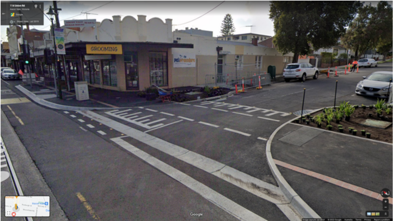
Raised asphalt platforms are different to continuous footpath treatments
