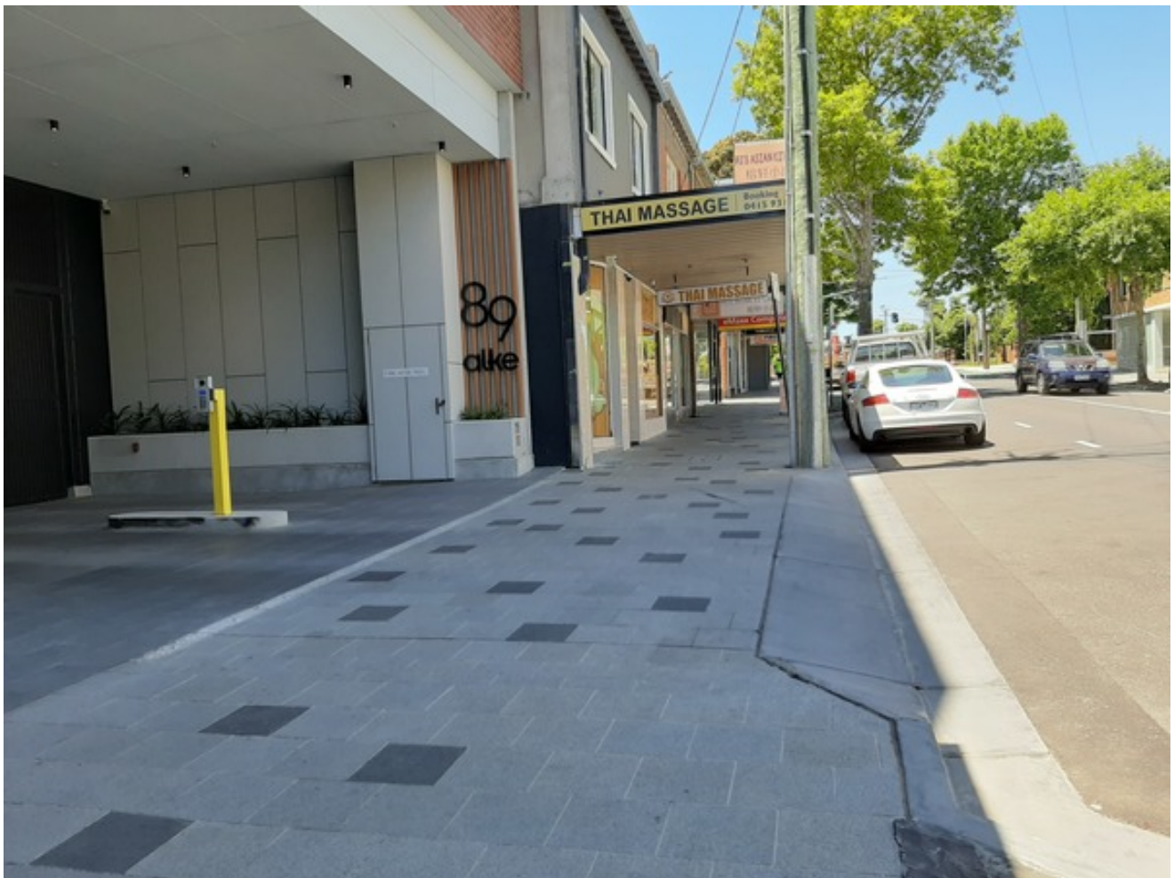
Continuous footpath design over driveway on Atherton Rd, Oakleigh
