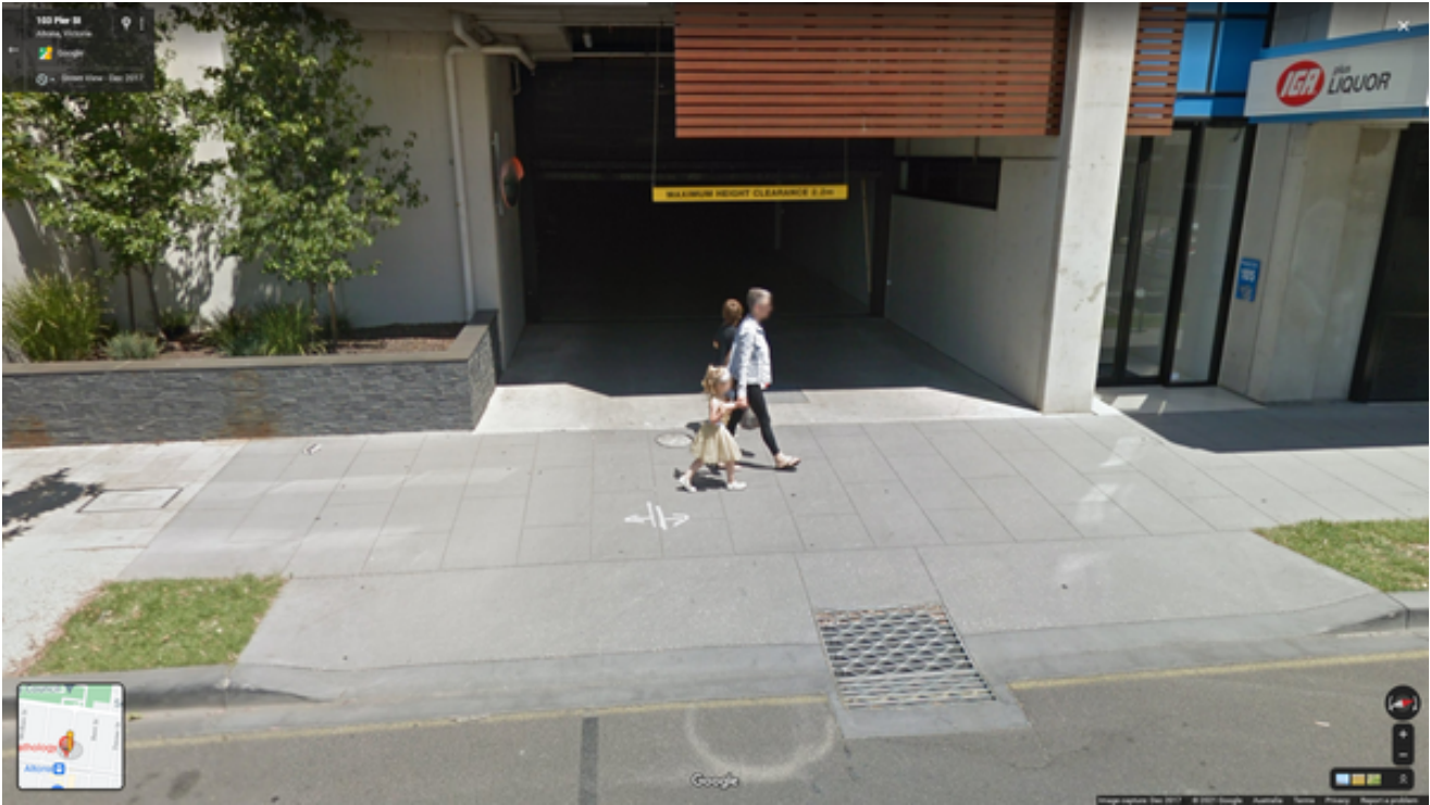
Continuous footpath made with stylised concrete
