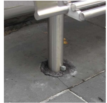
A seat installed into a gib key socket.
