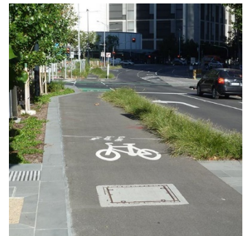
Raised separated bike lane
