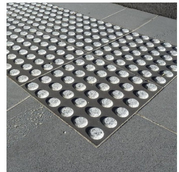
Examples of tactile paving
