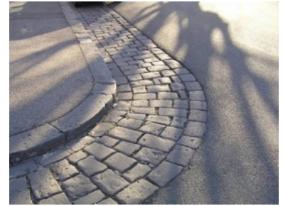
A traditional bluestone kerb and pitcher channel in North Melbourne. These add to the neighbourhood's character and heritage significance and should be conserved through timely maintenance and careful repairs when necessary that match the existing details.
