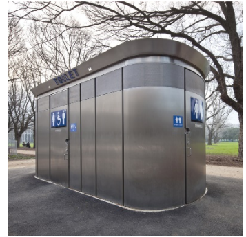
A typical self-cleaning toilet.
