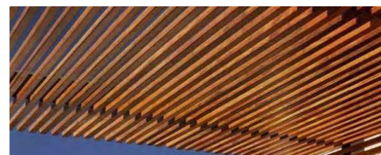
RFB EXPOSED DECORATIVE TIMBER ROOF BATTENS
