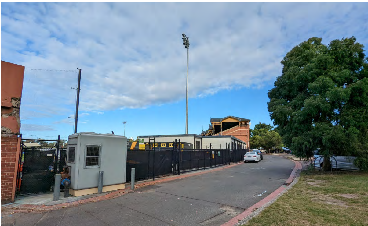
Site Photo of rear of Jack Dyer Stand and demountable buildings, showing vehicle access to above-ground car park and fencing/obstructing views into oval from Yarra Park (captured: 1 April 2022)
