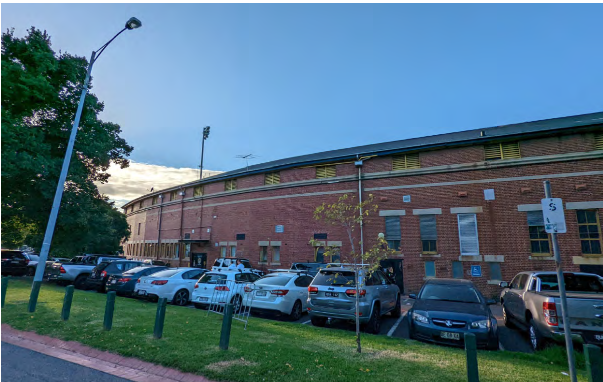
Site Photo of rear of Jack Dyer Stand showing curvilinear profile of grand stand and above-ground car parking (captured: 1 April 2022)
