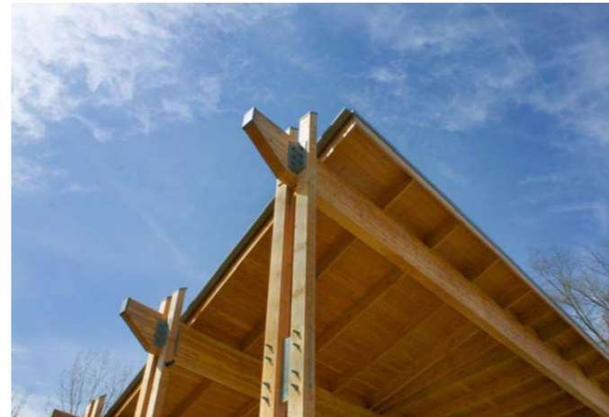
TFR RECYCLED TIMBER AS PRIMARY ROOF BEAM STRUCTURE
