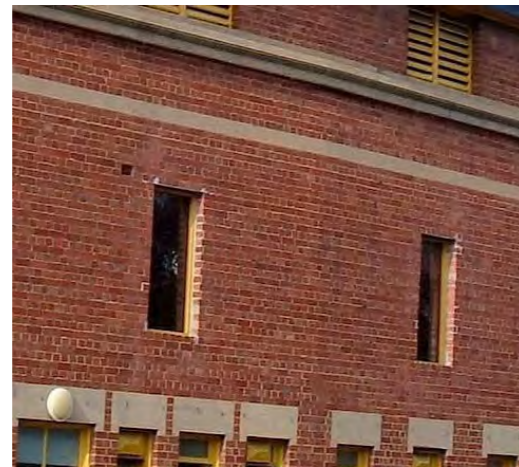
BR-01 RED BRICK RECYCLED FROM EXISTING JACK DYER WITH 'ENGLISH CROSS BRICK' PATTERN
