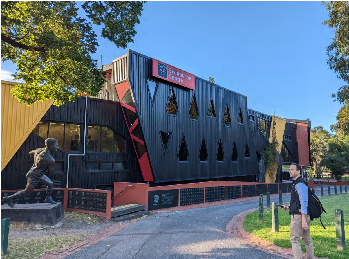
Site Photo of Swinburne Centre rear (west-facing) façade and Jack Dyer statue (note: person photographed is a CoM officer) (captured: 1 April 2022)
