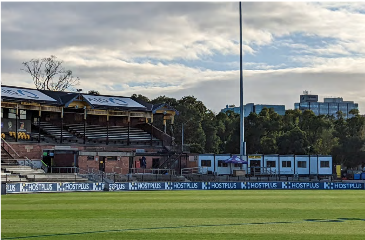
Site Photo of existing demountable buildings that will be removed/facilities consolidated in proposed development (captured: 1 April 2022)
