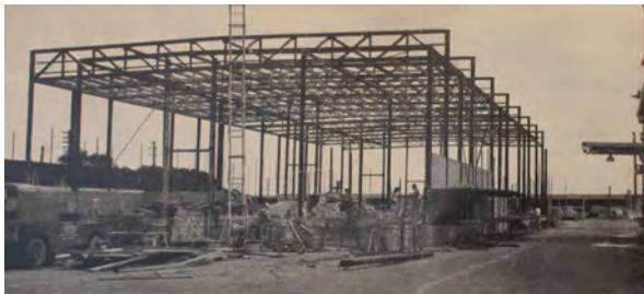
Figure 13: Cool room under construction in 1959-60, view from the north (Kraftsman, June-July 1960)
