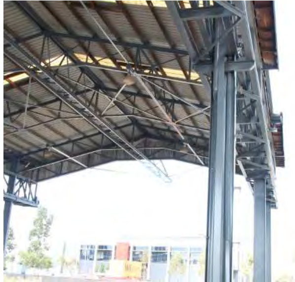
Figure 8: The tray, supported on the cambered part of the roof truss, still extends to the south over the truck loading bay and provides evidence of the electrical supply. Original light fittings are still evident. (P Mills, 03/04/2018)
