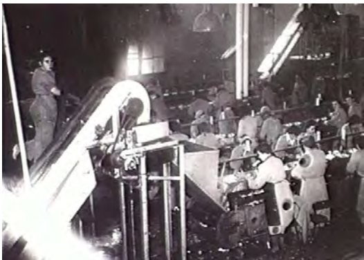
Figure 6: Women removing blemishes from peeled potatoes at the Kraft Walker-operated dehydration plant at Salmon Street, July 1945 (AWM photograph, Acc. No. 111137)
