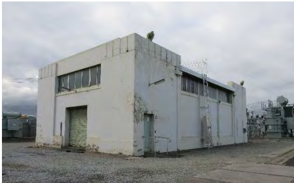
Figure 2: View of the substation from the southwest (H Lardner 09/07/2018)
