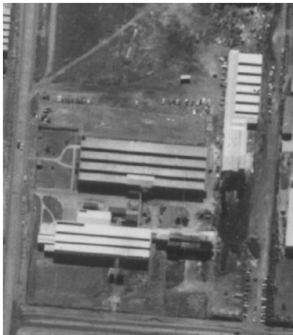
Figure 8: Extract of 1954 aerial showing the wartime dehydration factory, the 1945 yeast factory to the south east (Vegemite 'B'), and the three sawtooth bays of the new Vegemite factory. On the northeast the boiler house has been extended and the new workshops building (now part of Pilot Plant and Maintenance building) has been built further to the north (1954 aerial, Landata).
