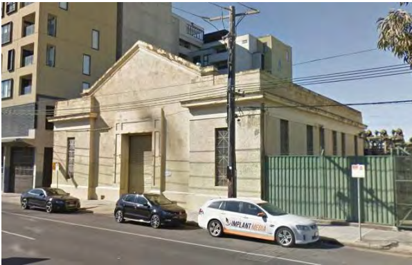
Figure 11: The SEC substation at 64 Brunswick Road Brunswick (Google image October 2017)
