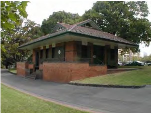
Figure 9: City of Melbourne c1940 pavilion-style Substation 5 at 2 - 4 Lansdowne Street East Melbourne (i-Heritage database)
