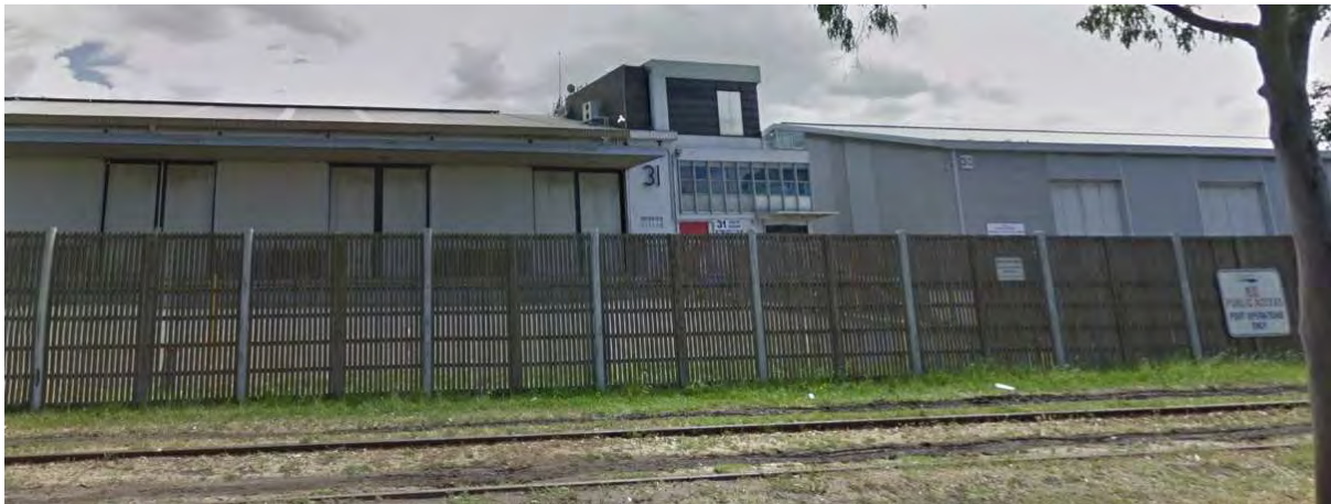
Figure 11: Shed 30 & 31, South Wharf at 593-629 Lorimer Street, Port Melbourne (Google imagery Oct 2017)
