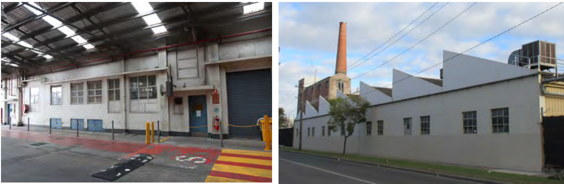
Figures 30 & 31: The west facade of the workshop building from under the covered way, and the sawtooth roof profile of east facade of the workshop building from Douglas Street. (P Mills 4/11/2020; HLardner 10/07/2018)
