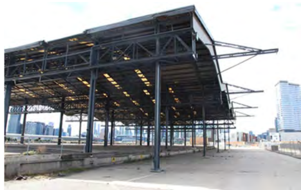
Figure 3: View from south-west showing road alignment and extension past the building. (P Mills, 03/04/2018)
