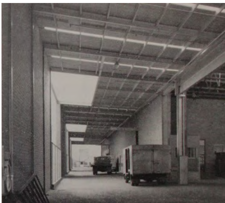
Figure 16: The new covered way on the west side, 1962 (Kraftsman, June-July 1962)
