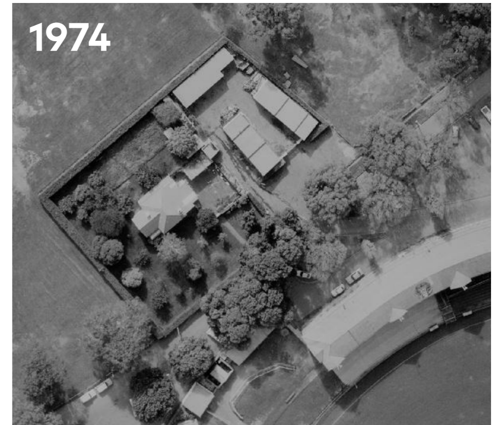
1974 Immediate environs used for parking. Caretaker's residence and works buildings later occupied by the Richmond Football Club.
