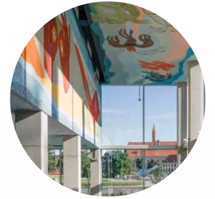
Feature ceiling to Atrium (printed metal)
