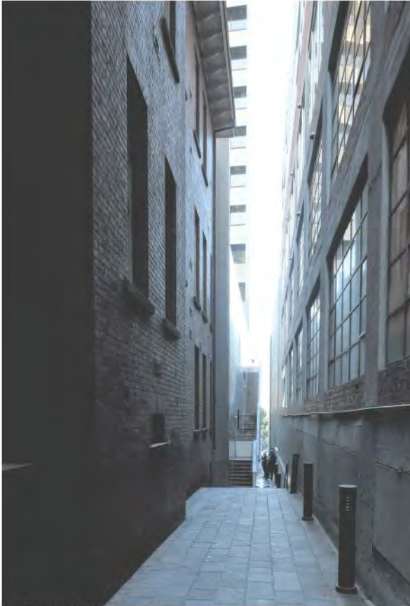
Existing Condition Western Laneway
