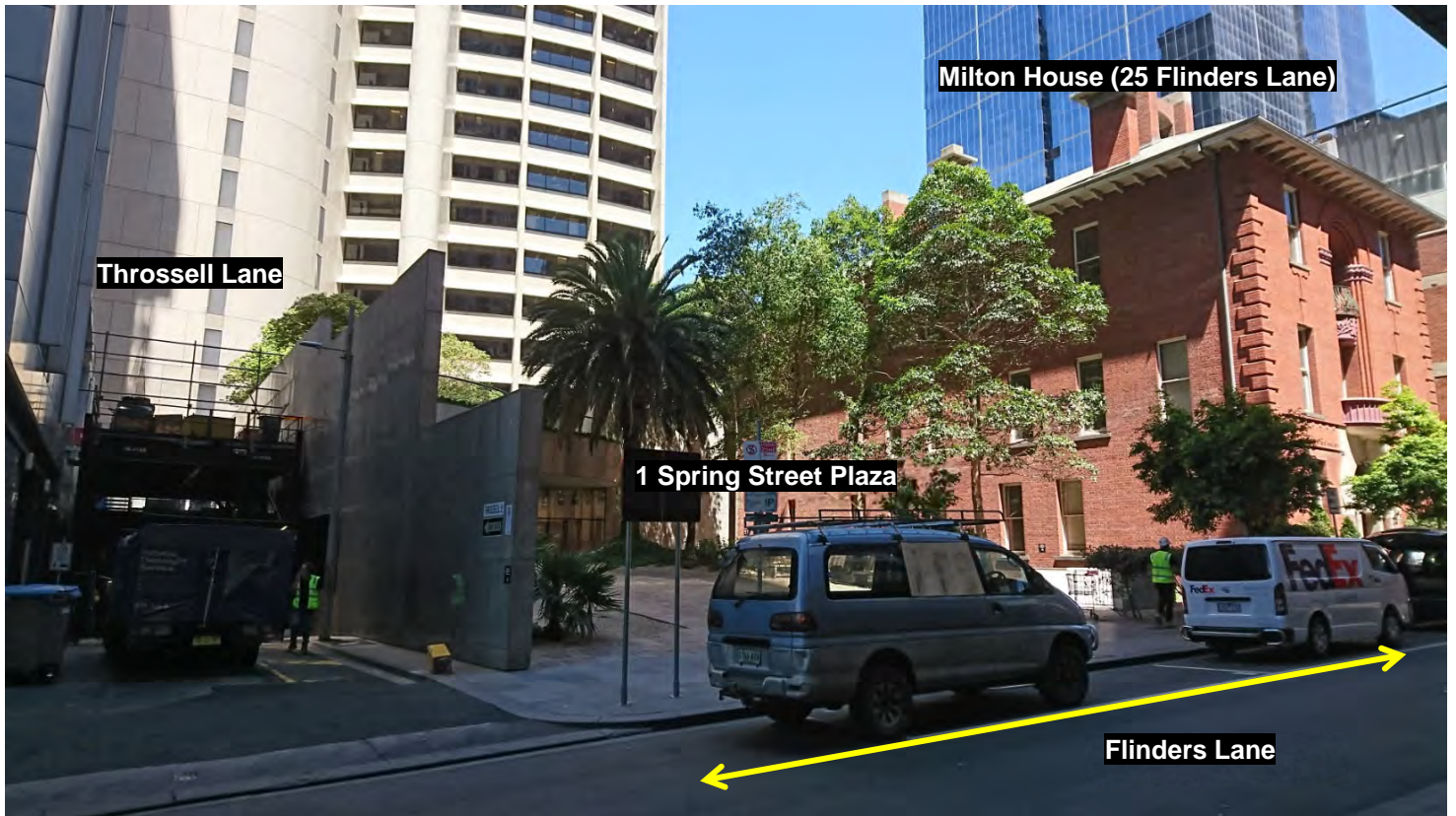
Flinders Lane frontage showing Throssell Lane scaffolding, captured: 27 October 2021
