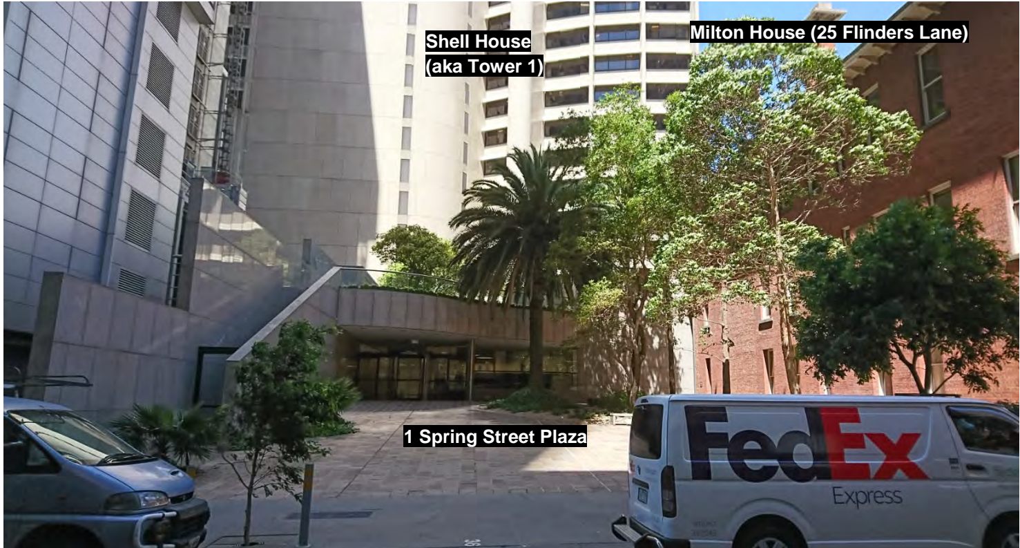
Flinders Lane frontage showing existing plaza adjacent to Milton House, captured: 27 October 2021
