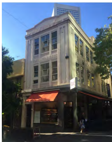
Figure 2 Farrant's Building, Source: Lovell Chen
