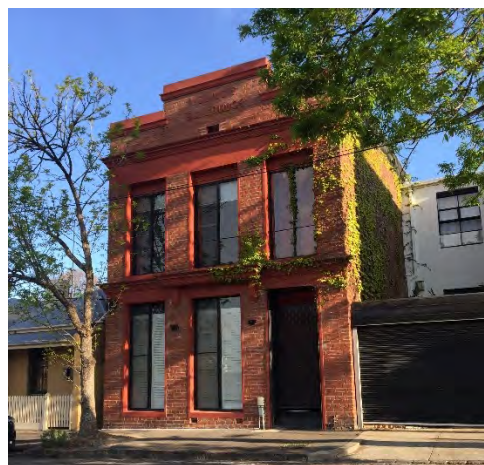
Figure 13 49 Owen Street, Carlton (HO1) Source: Lovell Chen
