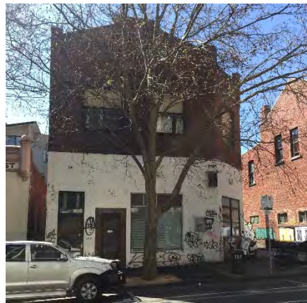
Figure 11 144-146 Queensberry Street, Carlton (HO807) Source: Lovell Chen
