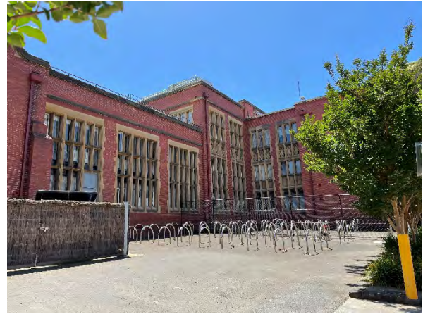
Figure 2 Peter Hall Building (HO820)
