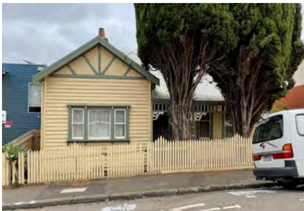
Figure 3 Residence, 2 Bayswater Road, Kensington (HO205)
