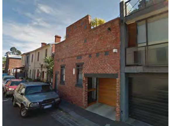
Figure 9 13-23 David Street, Carlton (HO1) Source: Streetview
