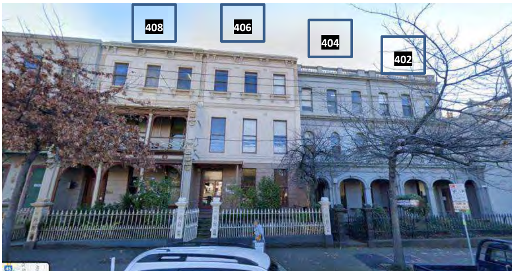
Figure 6 402-408 Albert Street, East Melbourne
