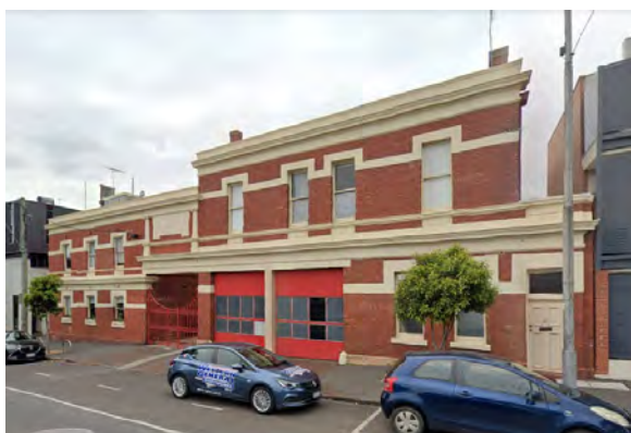
Figure 3 Former North Melbourne fire station, 100-110 Curzon Street, North Melbourne
