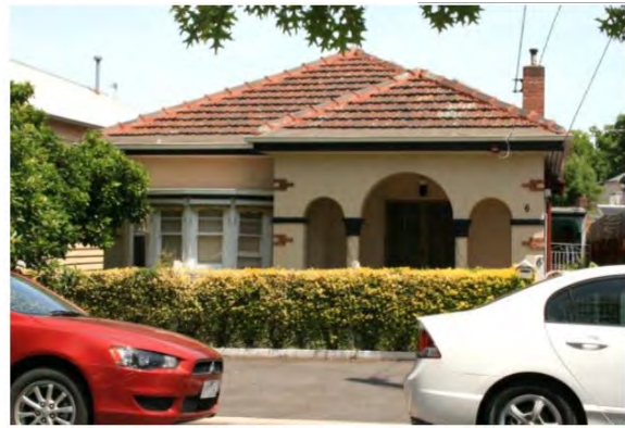
Figure 4 Waddington's houses, 6 Parsons Street, Kensington (HO1167)
