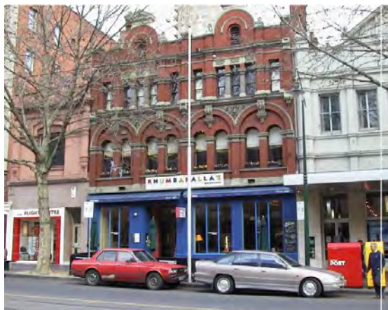
Figure 2 23-29 Bourke Street, Melbourne
