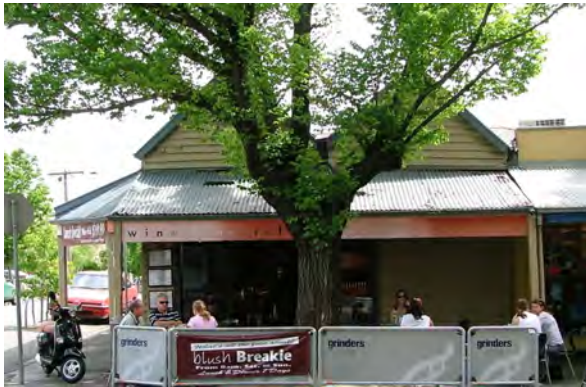
Figure 1 Shop, 43 Epsom Road (HO9) Source: City of Melbourne, via Hermes
