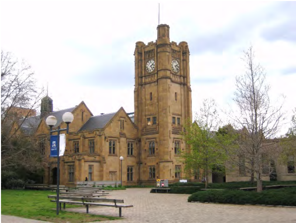
Figure 1 Old Arts Building (VHR 924)
