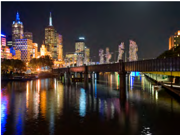
Sandridge Bridge is converted to a pedestrian and cycle path in 2006. It includes a major art commission – The Travellers by Nadim Karam – commemorating the bridge’s role as an entry to Melbourne for millions of migrants. [John Gollings]
