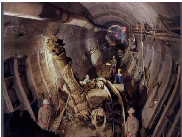
Following the 1969 Melbourne Transportation Plan, the City Loop was completed in 1978. This added an additional rail viaduct along the north bank. [John Holland Constructions, "The Loop" by Wolfgang Sievers, 1977. State Library of Victoria, Accession no: H2004.49/72]
