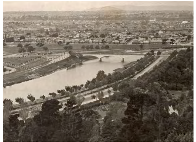
The river upstream is widened and straightened and treelined avenues built up along both sides. Part of the old channel is retained as the lake in the Botanic Gardens (right of image). The bend that was to the north of the Morell Bridge was filled (left of image). [State Library of Victoria]
