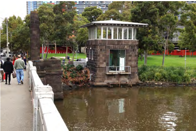
A structure formerly used to circulate water from the river to cool the Spencer Street power station is converted to a heliport office in 1996. This replaces a relocatable in Batman Park. [Ron Jones, City of Melbourne]
