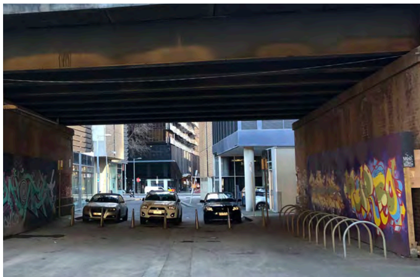
↑ ... unsafe, dark and noisy environments beneath the rail viaducts ...
