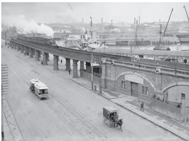
A viaduct is built between 1890-1894 linking Princes Bridge Station and Spencer Street Station. This is supported on a colonnade-like structure at the Turning Basin. The Banana Alley Vaults are built as part of this link. [State Library of Victoria]
