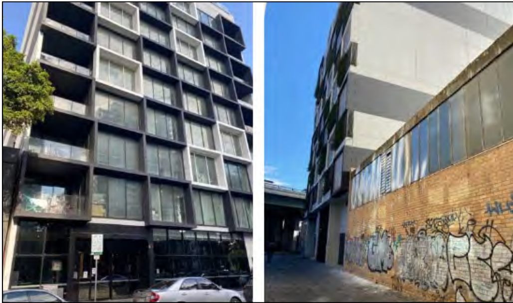
Figure 4: 63 Haig Street and Blakeney Place rear of the site (Source: Applicant)
