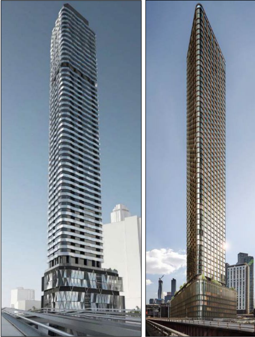
Figure 6 - Endorsed (left) and proposed (right) 3D render of the development, from Kings Way
