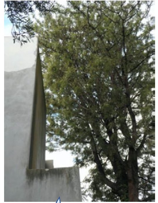
Unit 3 west wall
