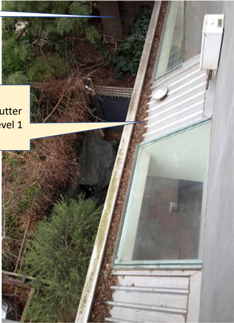
Photographs documenting leaves from tree 169 in gutters of units 4 and 3, 2019. – source: maintenance visits report to MBCM City owners corp managers
