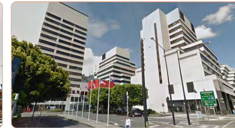
East Facade 02: The Eastern core is a prominent pivoting point in the original brutalist form. It anchors the site, and adjoins the main commercial entry. 4
