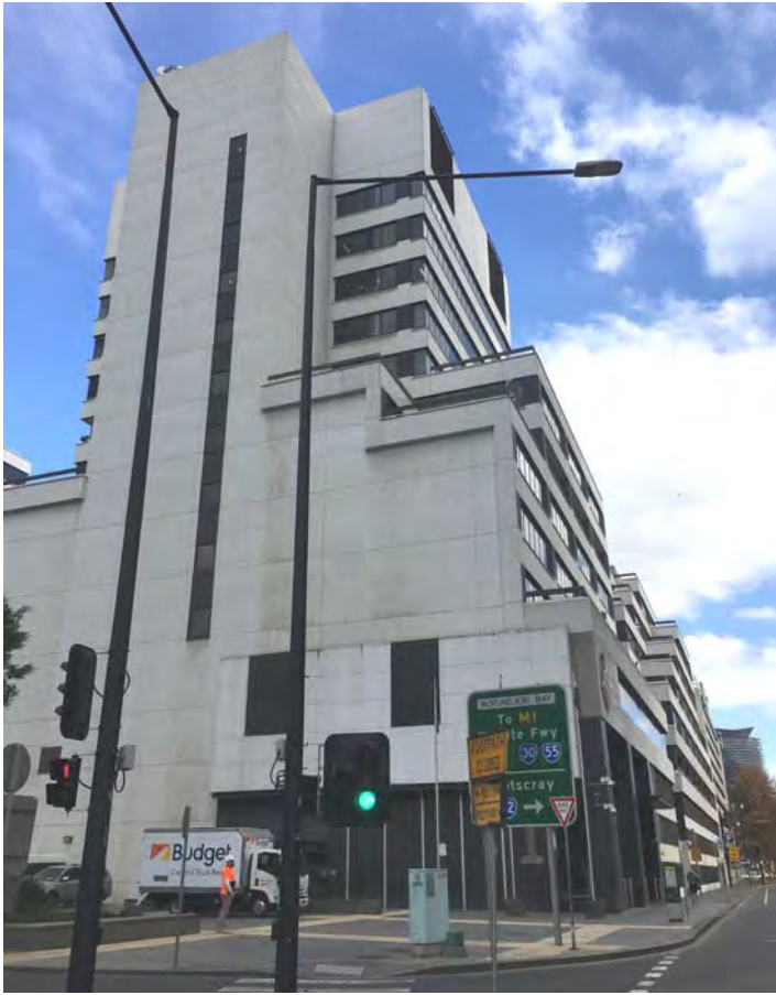
Figure 2 - View of site from the north-east, along Flinders Street
