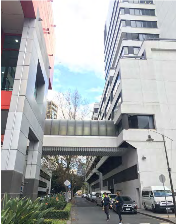
Figure 2 - View west along Siddeley Street, with subject site on right
