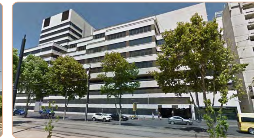
North - West Facade: The view highlights the aggressive nature of the Flinders St frontage, with heavily vehicle traffic. 2
