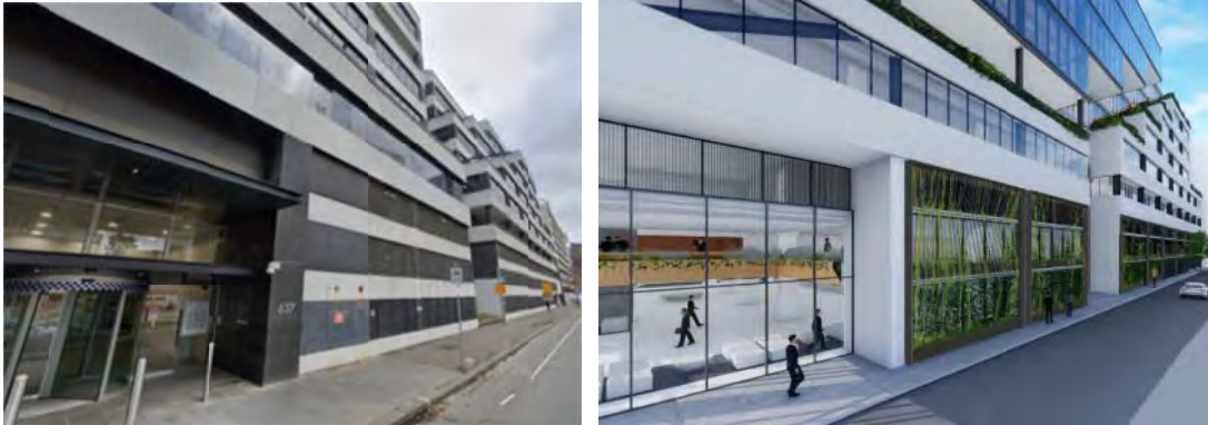
Figure 13 – Street view image of existing building (left) and 3D render of proposed ground level
