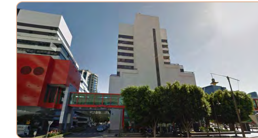
East Facade 01: Discussions are ongoing between surrounding precinct owners around the worth of and desire to remove the red box and bridge link. 3
