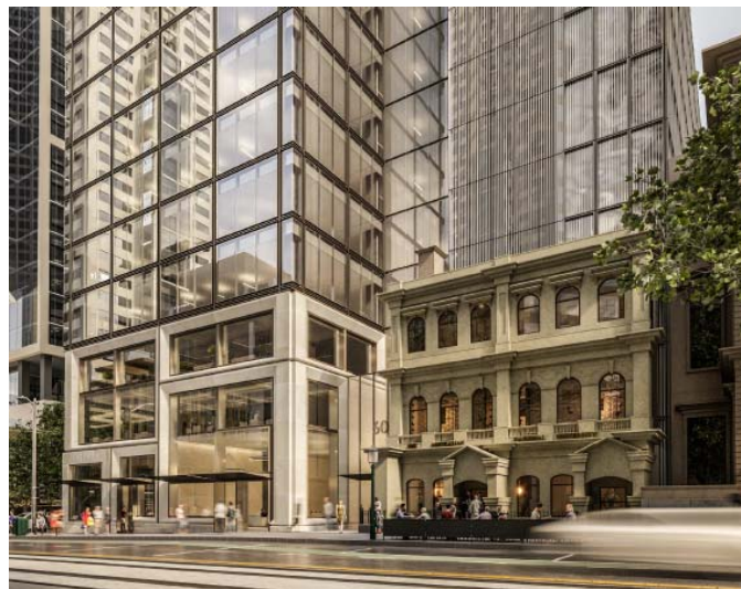
Figure 5: Ground level treatment of building as viewed from Collins Street (source: Bates Smart submitted architectural plans)
