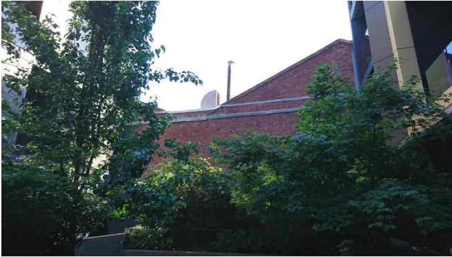
Figure 1: Current North boundary wall of 68 Leveson St
