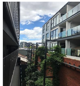
Figure 4: Alternate view from L3 to East boundary wall
