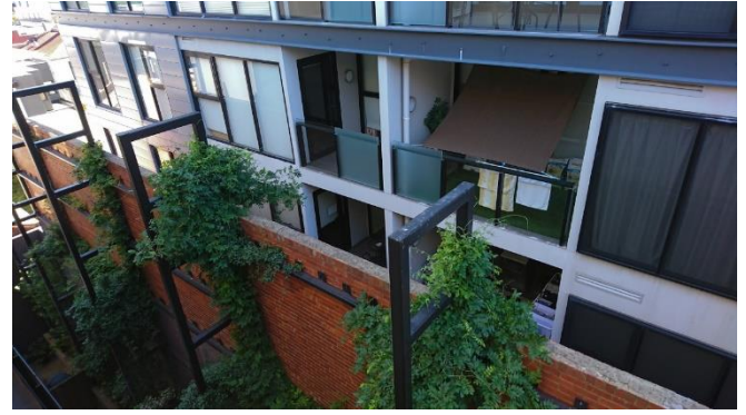
Figure 2: Current East boundary wall of 68 Leveson St
