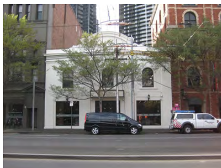
107-127 Queens Bridge Street (part) – proposed HO1200 (former Castlemaine Brewery) contributory to proposed HO1214, interim HO1200 applies
