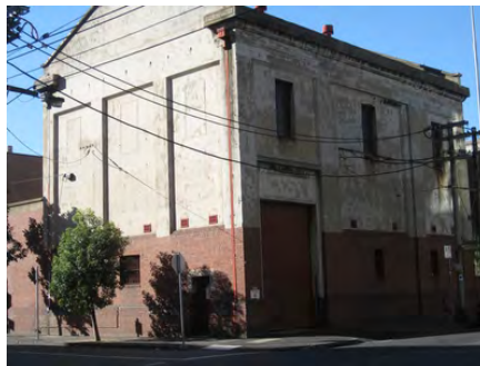
67-69 Clarke Street – proposed HO1223 (Melbourne Metropolitan Tramways Board Electricity Substation 'S'), contributory to proposed HO1214
