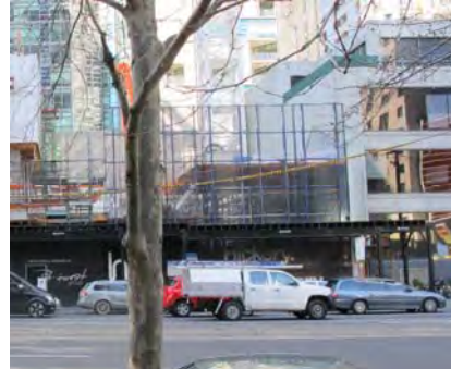
43-47 City Road – contributory to proposed HO1214 (City Road Industrial and Warehouse Precinct)
