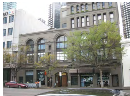
107-127 Queens Bridge Street (part) – proposed HO1229 (Robur Tea Company factory-warehouse), contributory to proposed HO1214
