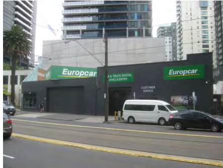
56-62 Clarendon Street – contributory to proposed HO1214 (City Road Industrial and Warehouse Precinct)
