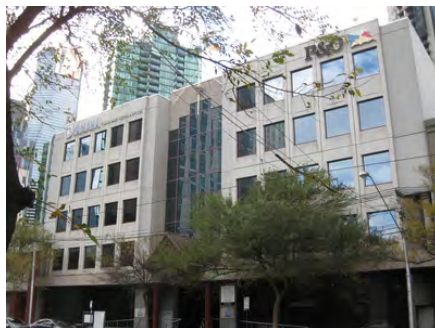
99 Queens Bridge Street – not a proposed heritage place
