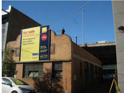
11-13 Hancock Street – contributory to proposed HO1214 (City Road Industrial and Warehouse Precinct)
