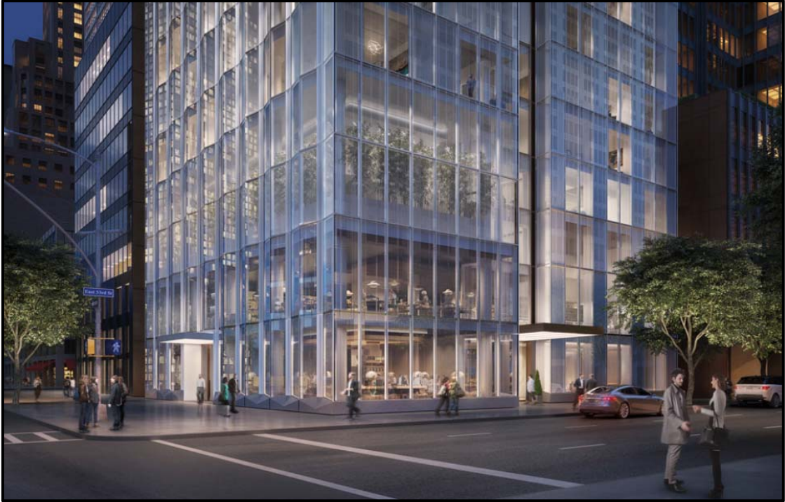
Excerpt from render of tower base as originally proposed in application received by Council on 15 December 2016
