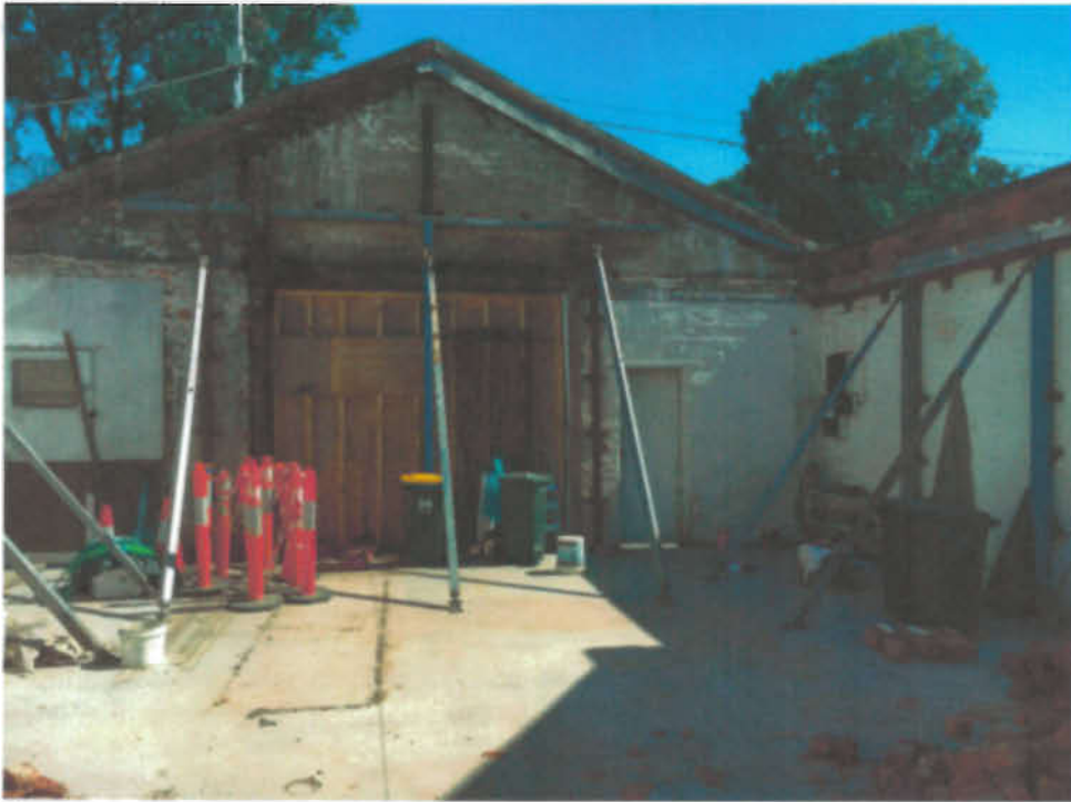
View of inside of west wall.
