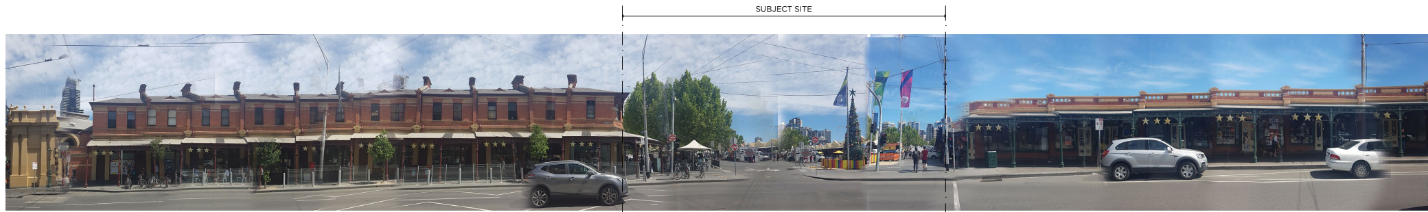
01 Victoria Street Facing South
