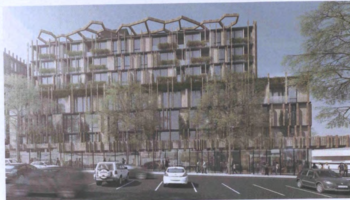
01. BUILDING A ROSSLYN ST. VIEW
