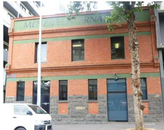
139-141 Franklin Street, Melbourne (C Graded)
