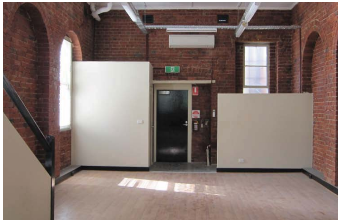
A. Internal elevation, rear exit door to external stair
