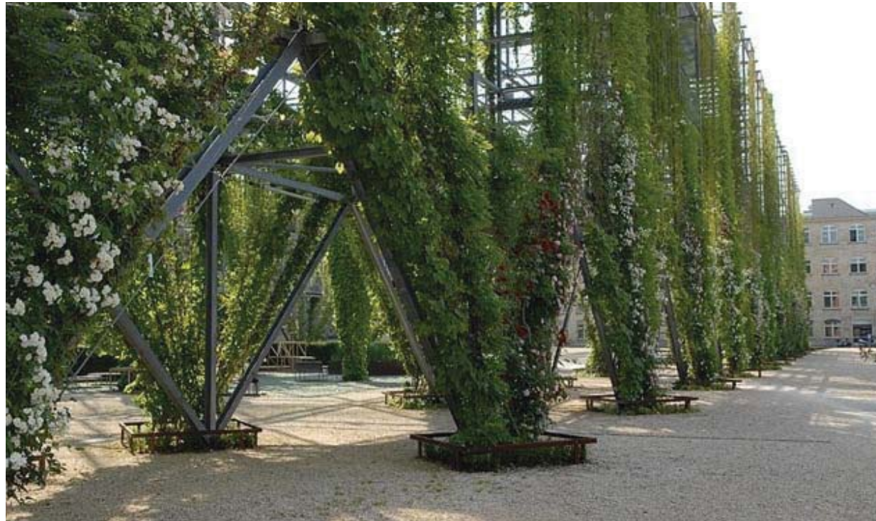
Vertical planting attached to metal frame structure, MFO Park Zurich
