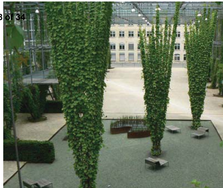
Vertical planting attached to metal frame structure, MFO Park Zurich
