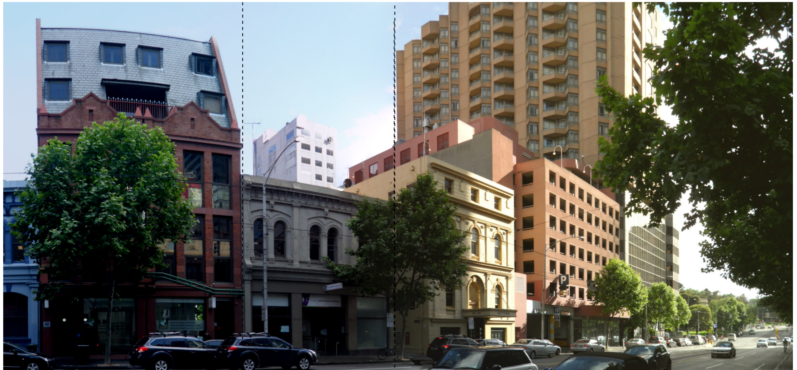
NO. 40 LATROBE STREET VIEW FROM MACKENZIE STREET
