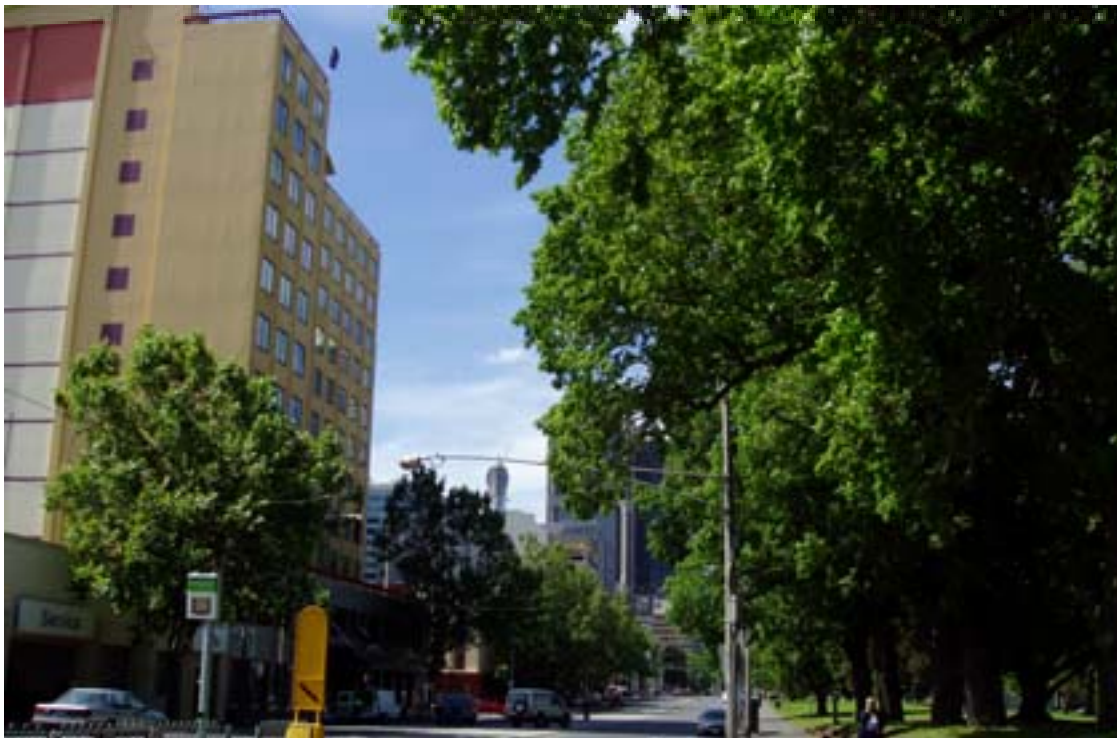
Photo 8 Relationship between the Radisson Hotel and eastern edge of Flagstaff Gardens (shadows as at mid morning in mid November)
