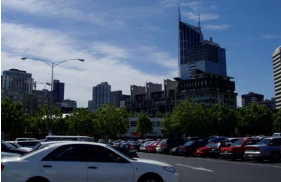
Photo 9 View across QVM car park towards Melbourne Terrace (32.4m) on the corner of Queen and Franklin Streets with higher buildings in Central Activities District behind.
