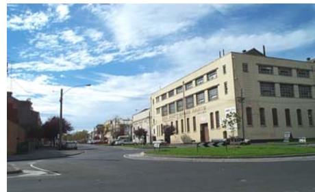
Warehouse buildings in West Melbourne Example of a Precinct undergoing change.
