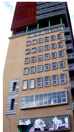
Residents will occupy both converted commercial buildings and new purpose-built apartment towers in the CBD and along St Kilda Road .
