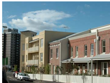
Public housing development, Kensington There is opportunity for the renewal of many of the Inner Region's public housing estates.
