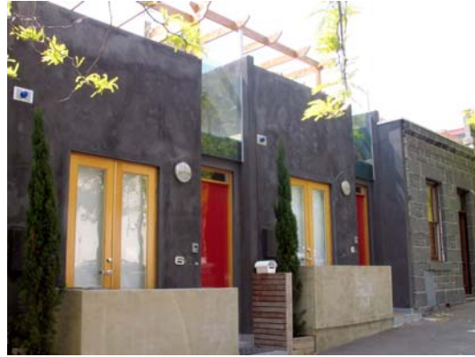
Courtney Street, North Melbourne
