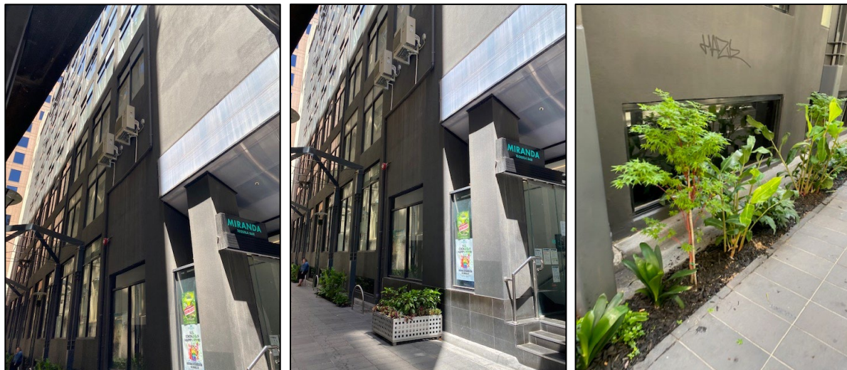
Figure 5 – Views of Mill Place and windows projecting from basement which include soundproofing / blackout (far right) (taken 13 November 2023)
