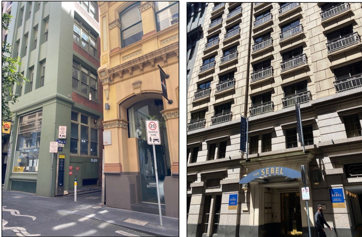
Figure 4 – 310 Flinders Lane (left) and 302 Flinders Lane (Leicester House) (right) on the corner of Flinders Lane and Bligh Place and The Sebel located to west of the subject site (taken 13 November 2023)
