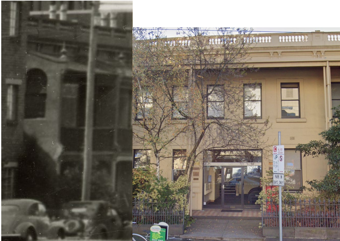
As Above: Photo showing the 1883 verandah taken in 1950/59 (Left) (Source: SLV) and Photo of existing verandah (Right) (Source: Google Streetview 2019)
