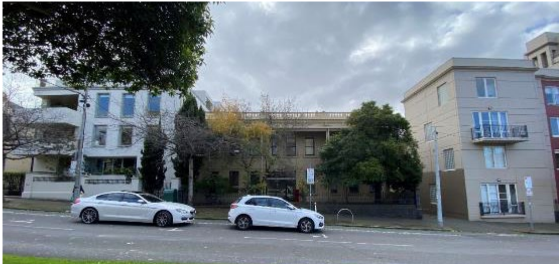
As Above: The Site and adjoining properties as viewed from Albert Street (Captured 1 June 2023)
