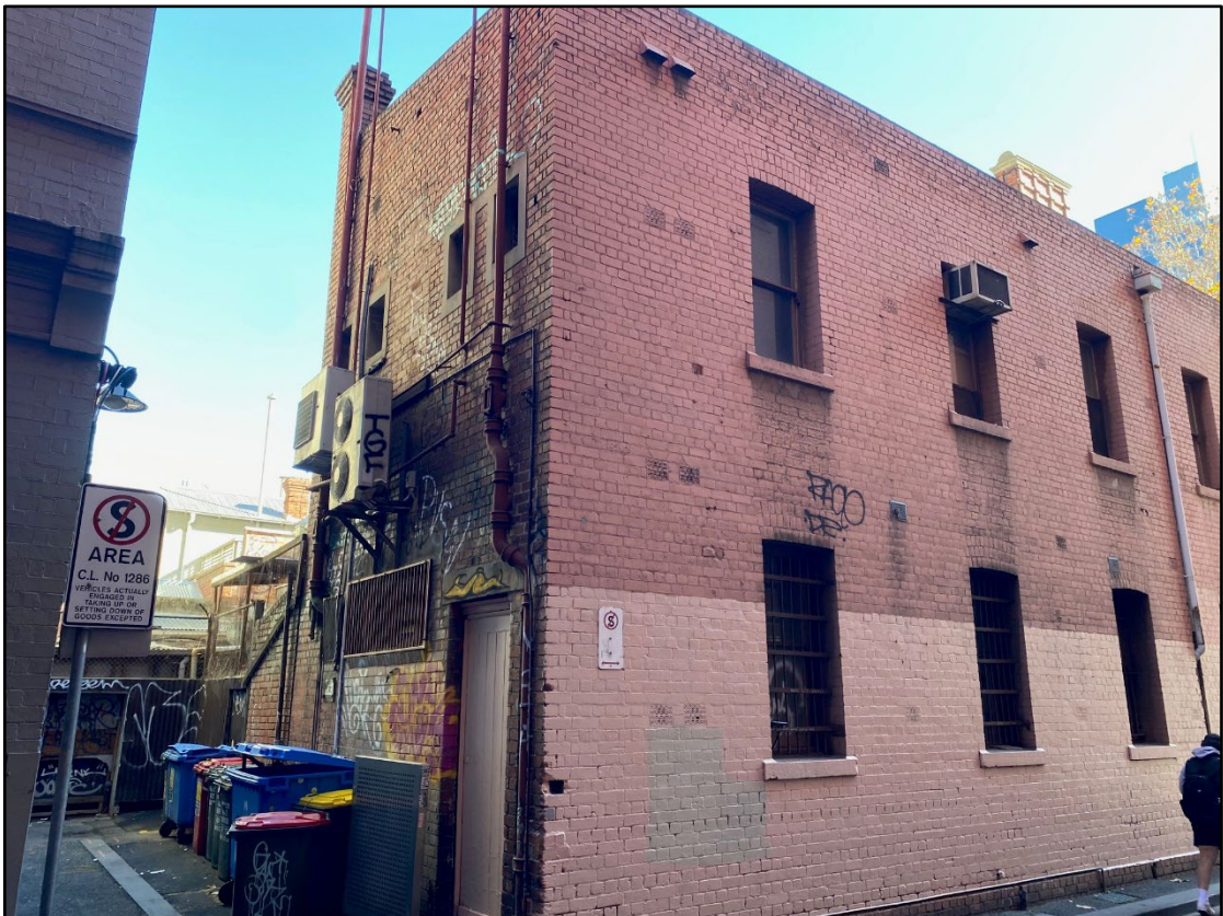
Figure 4: Rear Elevation of 19-21 Bourke Street (Council Lane, photograph taken prior to commencement of demolition works)
