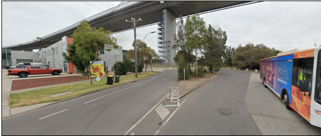
Figure 5: View from the south along Lorimer Street
