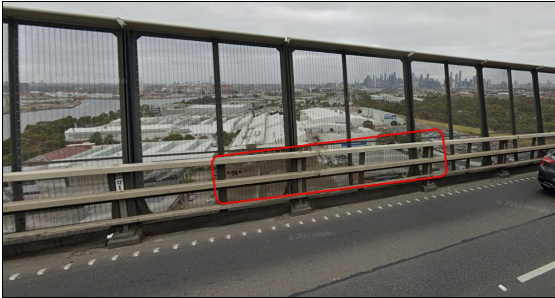
Figure 2: View of Site from Westgate Bridge
