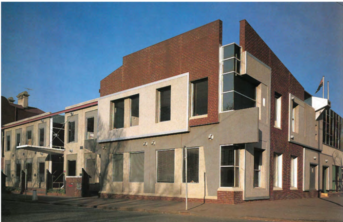
Figure 5 The subject building, photographed in 1994 Source: Graham Jahn, Contemporary Australian Architecture , Gordon and Breach Arts International, Sydney, 1994, p. 113
