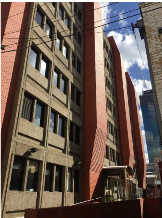
Figure 6 Detail of rear or north elevation of Building 51, with massive brick pilasters or shafts Source: Lovell Chen
