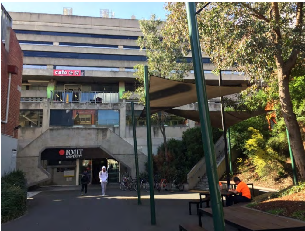
Figure 14 South façade of Building 57, as seen from O'Grady Place, with concrete tiered levels and concrete entrance ramp Source: Lovell Chen
