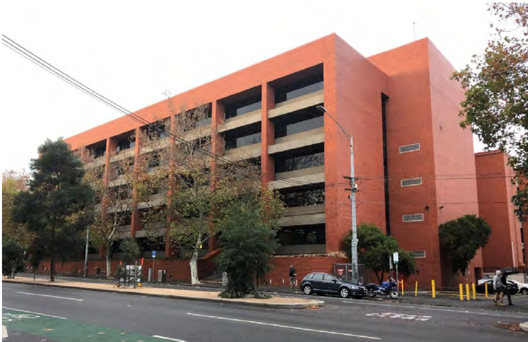
Figure 8 Building 56, north façade, as seen from Queensberry Street; the entrance is via the steps at centre image Source: Lovell Chen
