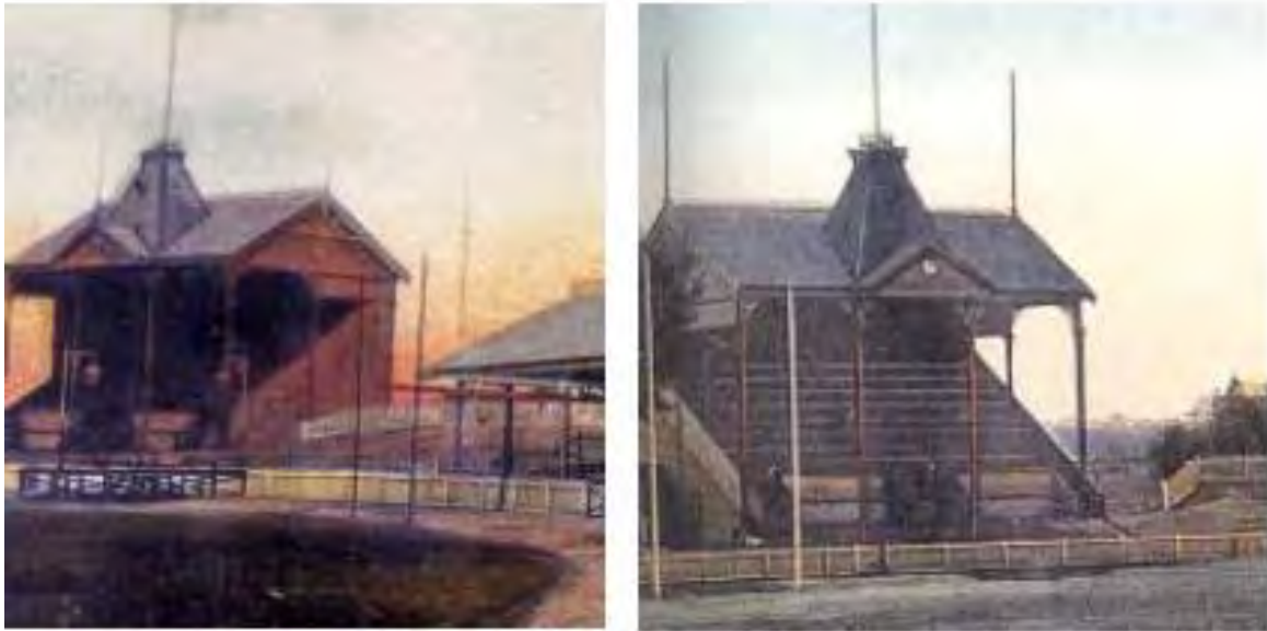
Figure 3. Small stand at Victoria Park (demolished) designed by William Pitt, built 1892. (Source: State Library Victoria (left) and McFarlane and Roberts 1999 (right), from Allom Lovell & Associates 2003: 60)
