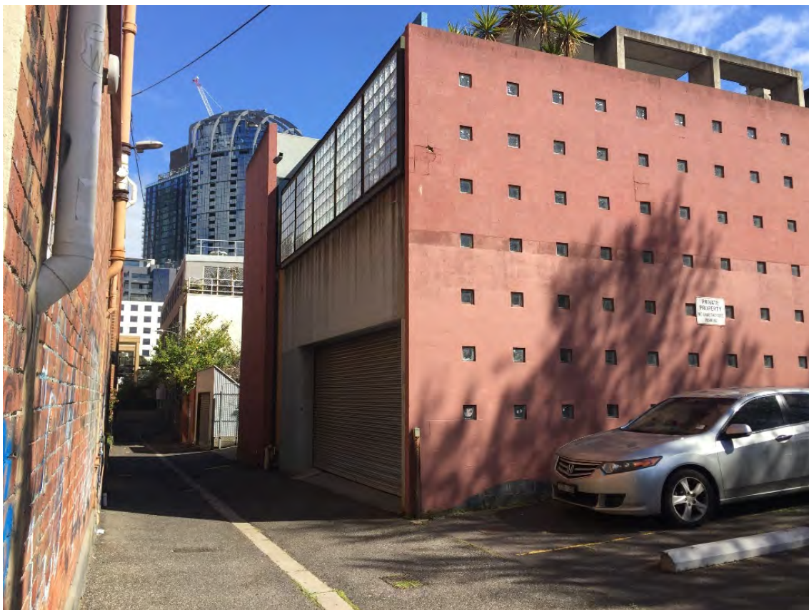
Figure 4 Looking south along rear lane, with the 'perforated' Queensberry Street elevation at right Source: Lovell Chen
