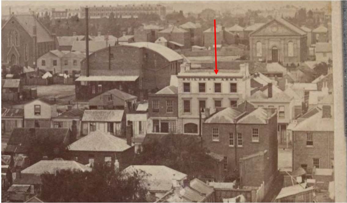
Figure 3 View of Carlton between Queensberry and Victoria streets in 1870, looking east past Cardigan Street towards Carlton Gardens in the distance, 1870. Subject site indicated Source: Charles Nettleton, photographer, H96.160/1433, State Library of Victoria
