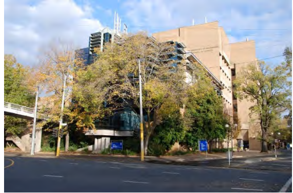
Figure 18 David Caro Physics Building, University of Melbourne (1970-73) Source: Film Victoria
