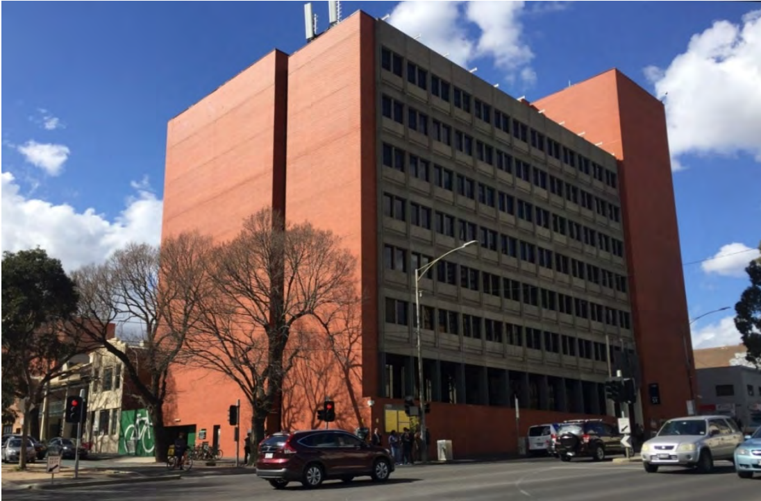
Figure 5 Building 51 as viewed from the corner of Victoria and Cardigan streets; the concrete façade faces south, with the service tower and stepped entry at the east end (right of image); the brick elevation at left faces west Source: Lovell Chen
