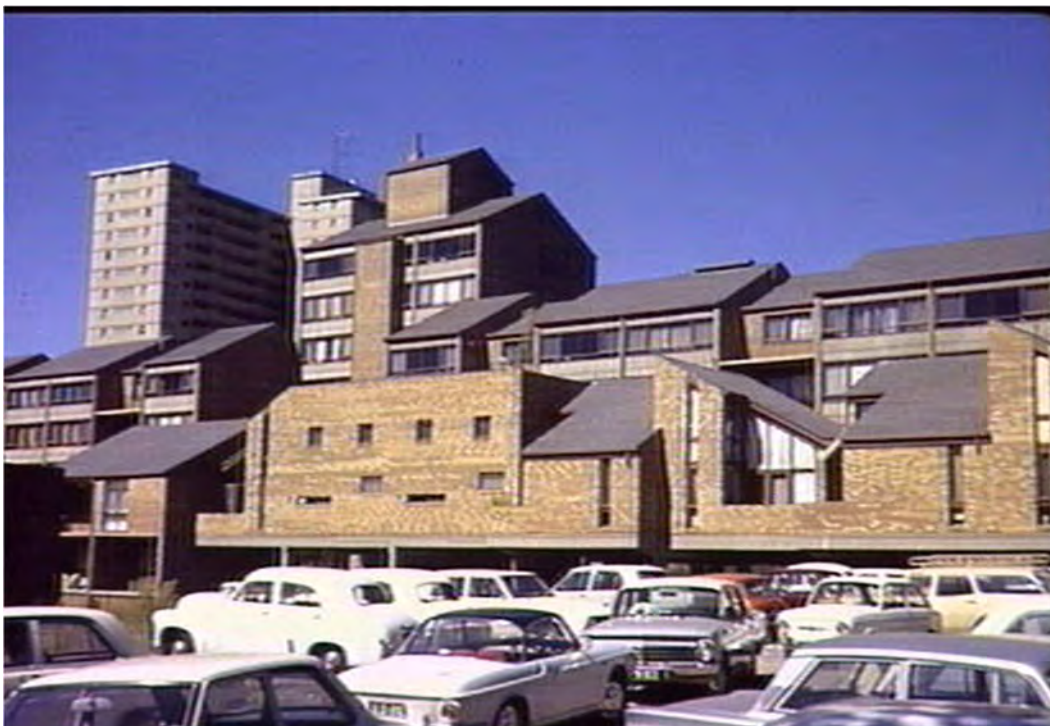
Figure 9 Completed Cross Street Co-operative Development, Lot 1, 1970 Source: Peter Wille, H91.244/1839, State Library of Victoria Picture Collection
