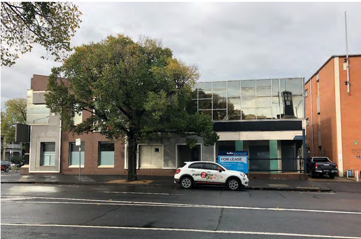
Figure 9 Grattan Street elevation of subject building Source: Lovell Chen
