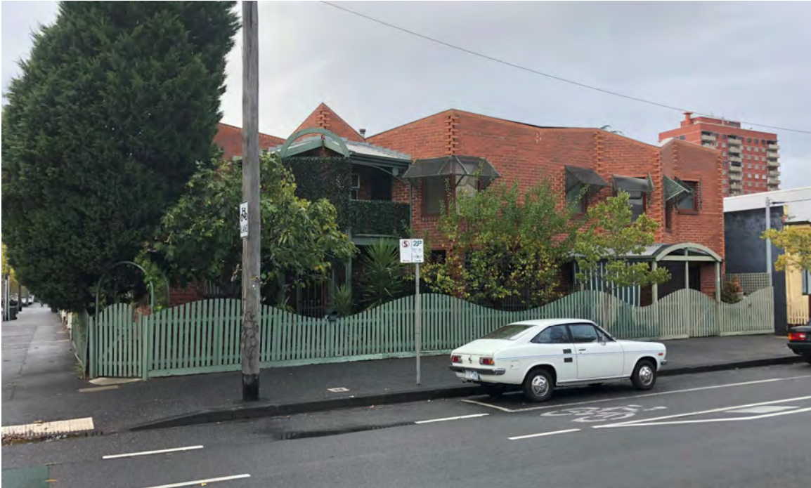
Figure 10 43-45 Kay Street and 136 Canning Street (Gregory Burgess) Source: Lovell Chen
