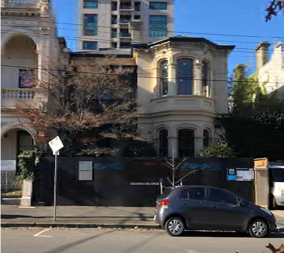
Figure 5 Victorian villa, 64-68 Drummond Street, Carlton
