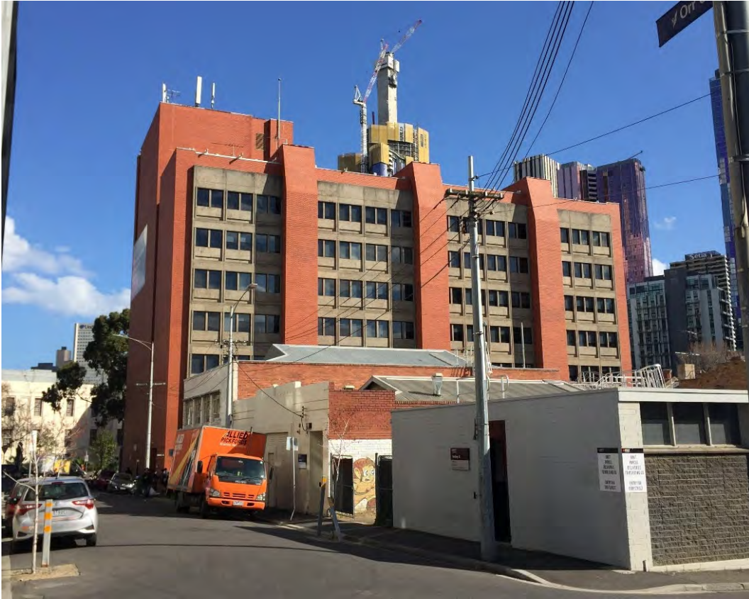
Figure 7 North side of Building 51, as seen from Earl Street Source: Lovell Chen
