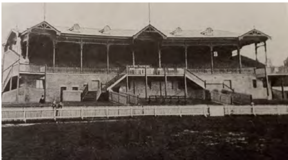
Figure 28. Early image of the grandstand (Jack Dyer Stand) at Punt Road Oval, built 1913–14 to a design by Thomas Watts & Son (shown here before the 1927 extension to the west). (Source: Hansen 1989: 34)
