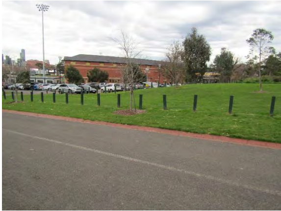
Figure 22. View to the rear of the Jack Dyer Stand approaching from Yarra Park (northeast). (Source: Context-GML 2021 )
