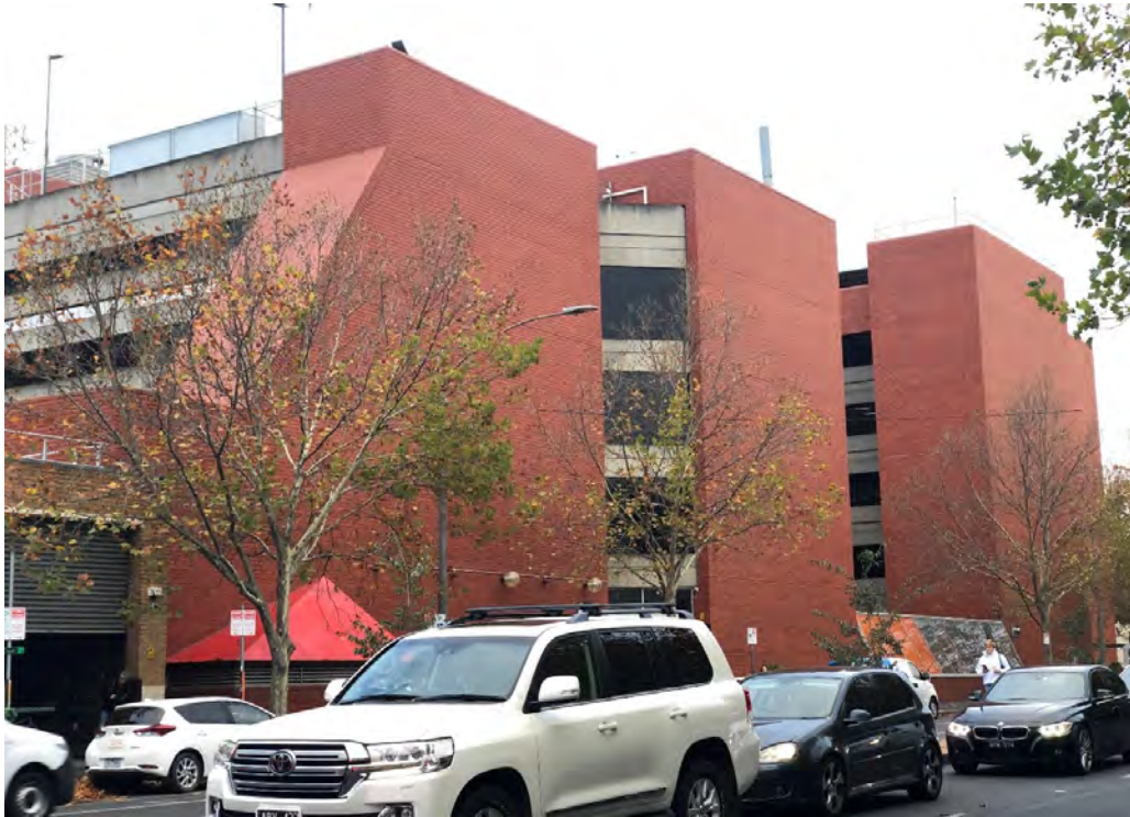
Figure 15 Buildings 57 and 56, as seen from the south on Lygon Street; note the tiered form of the south elevation of Building 57 (at left) Source: Lovell Chen
